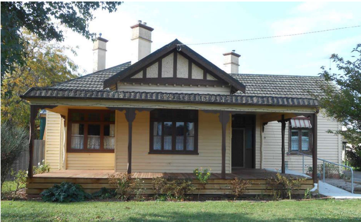
Figure D7. St John's Rectory to the north-west of the church is a large weatherboard residence with a complex hip-and-gabled roof clad in tiles, with exposed rafter ends to the eaves. The facade has a central projecting gabled-bay with rough-cast render and timber strapping to the gabled-end, creating a half timbering effect. ( L Barraclough 2016)
