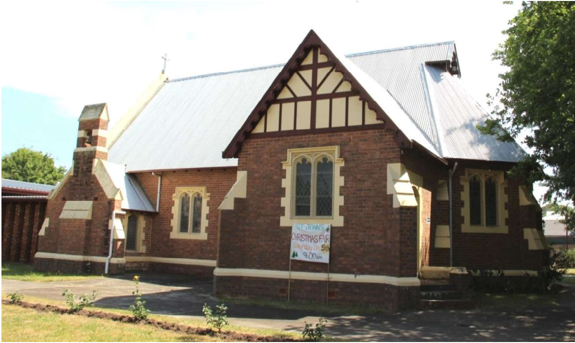
Figure D2. To the right, the south-east elevation has a flying gablette off the ridge, above the projecting bay of the chancel end with Queen Anne architectural detailing.
