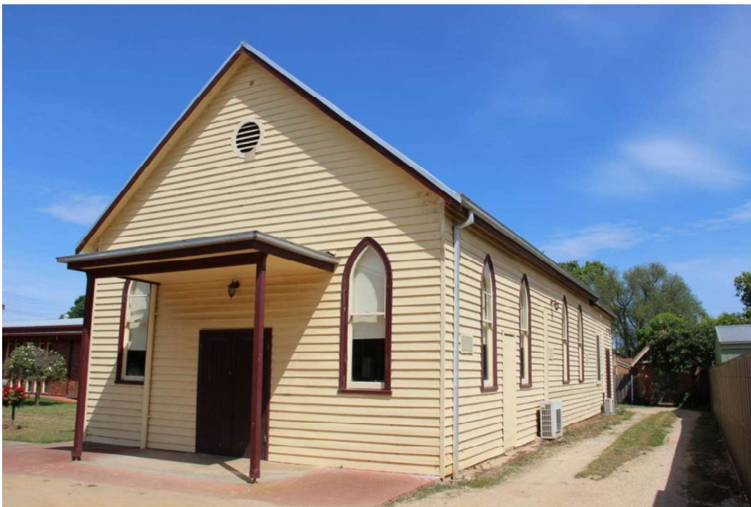
Figure D5. To the north of the church is the 1889 weatherboard hall. The long building has a gabled-roof clad with (recent) corrugated iron with a gabled end fronting Thomson Street, with pointed-arch windows.
