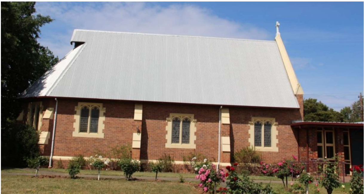
Figure D3. The north-east elevation comprises three bays, broken up by buttresses with rendered coping. Each bay has a pair of windows in the same detail as the rest of the church.
