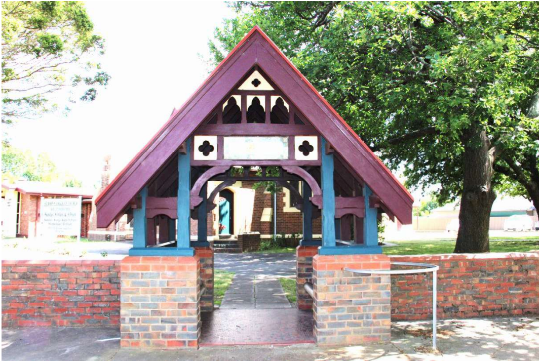
Figure D8. A picturesque Interwar Arts and Crafts, gabled-roof lych gate is located at the southern corner to the property. The roof is clad with slate and supported by posts with ornate timberwork with Gothic-inspired foil motifs. Adjoining the gate are the brick columbarium, which holds a number of plaques, and memorial brick fence with mild-steel railings.
