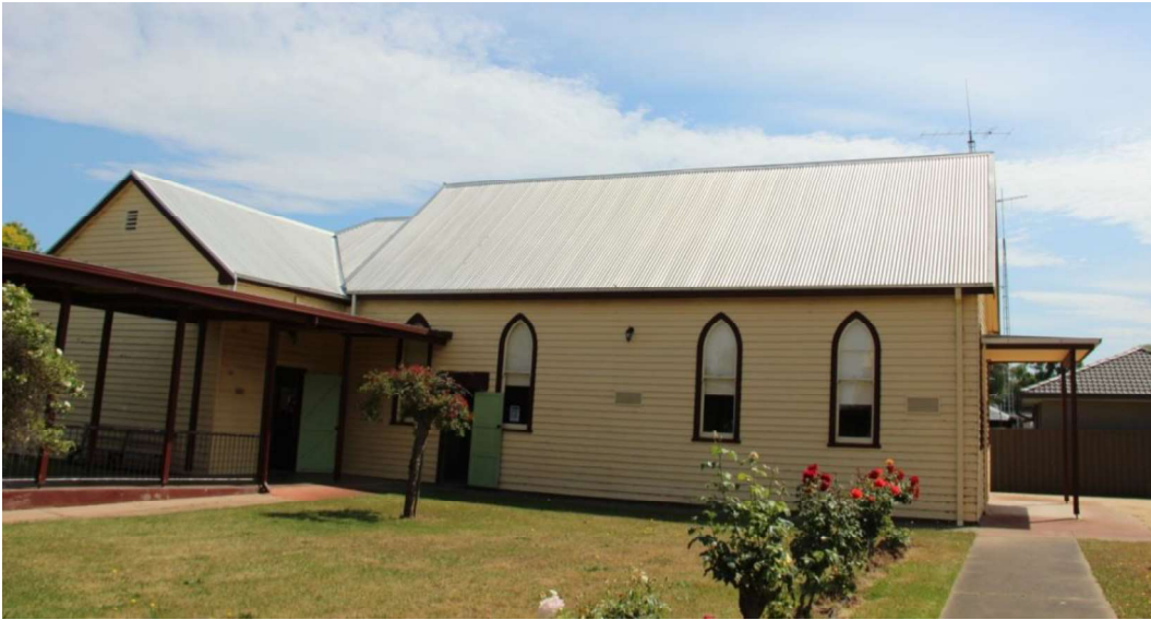
Figure D6. The side elevations of the church have four tall windows, and one or two doors on each side. To the rear of the church is a smaller weatherboard addition with a transverse gable.
