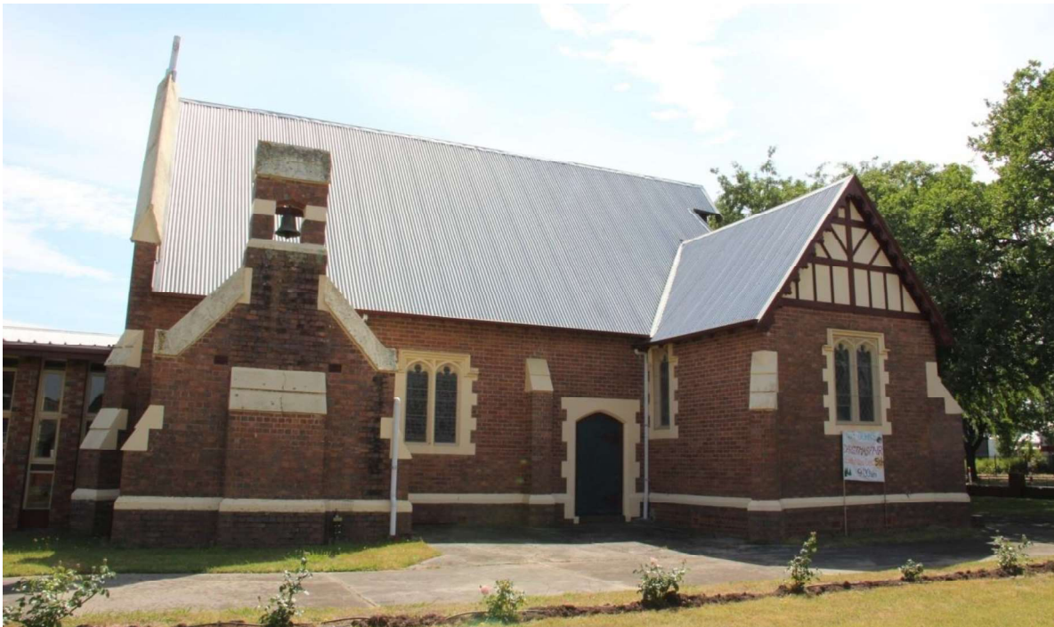
Figure D1. The brown brick church (1900) reflects the Federation Gothic style. It's steeply pitched gabled-roof is clad with (recent) corrugated iron and has a parapeted gabled to the north-west elevation. The south-west elevation fronting church street has the bellcote at the left end, which a parapeted gable and the details of the nave. To the right is the large gabled-end of the projecting entrance porch with the timber strapping forming a cross.
