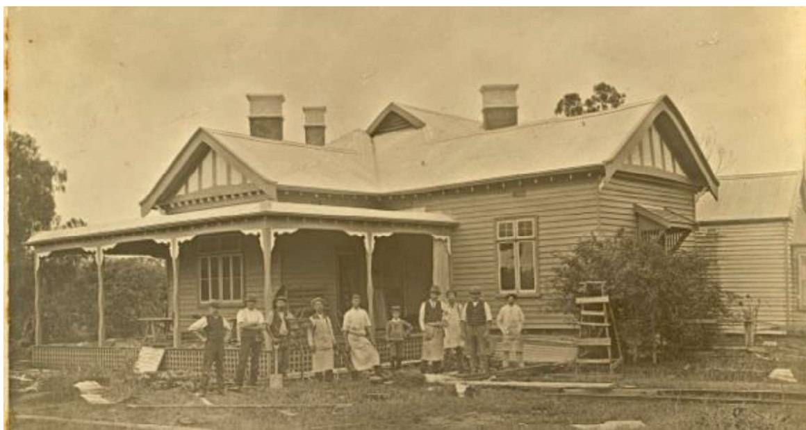
Figure H7. A 1912 photo of the almost-finished Anglican rectory at Maffra in 1912. A sign can be seen that notified that the building was being constructed by Alex Hardie, a well known Maffra builder (MDHS, ID. P04767VMFF).
