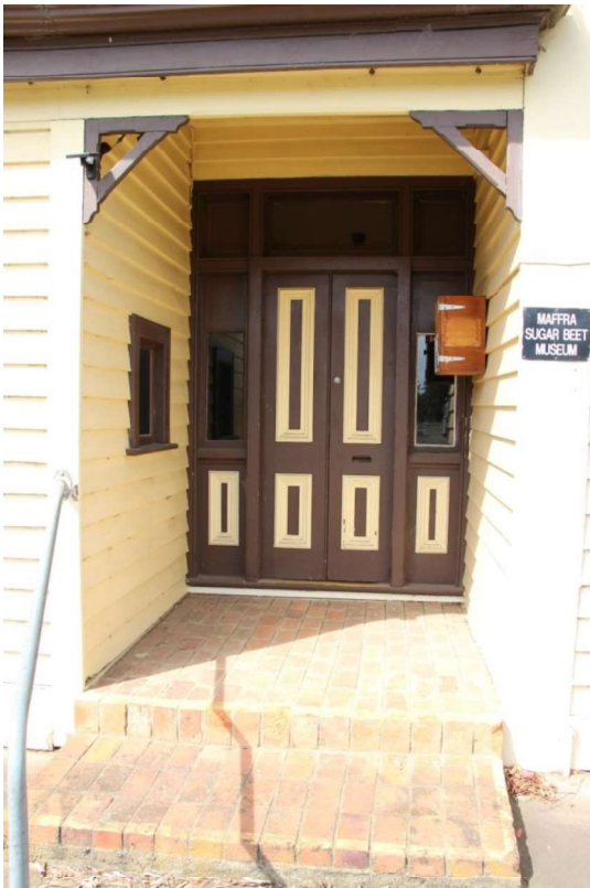
Figure D2. The recessed entrance to the office, with its simple timber brackets and the pair of panelled timber doors, with highlights and sidelights.
