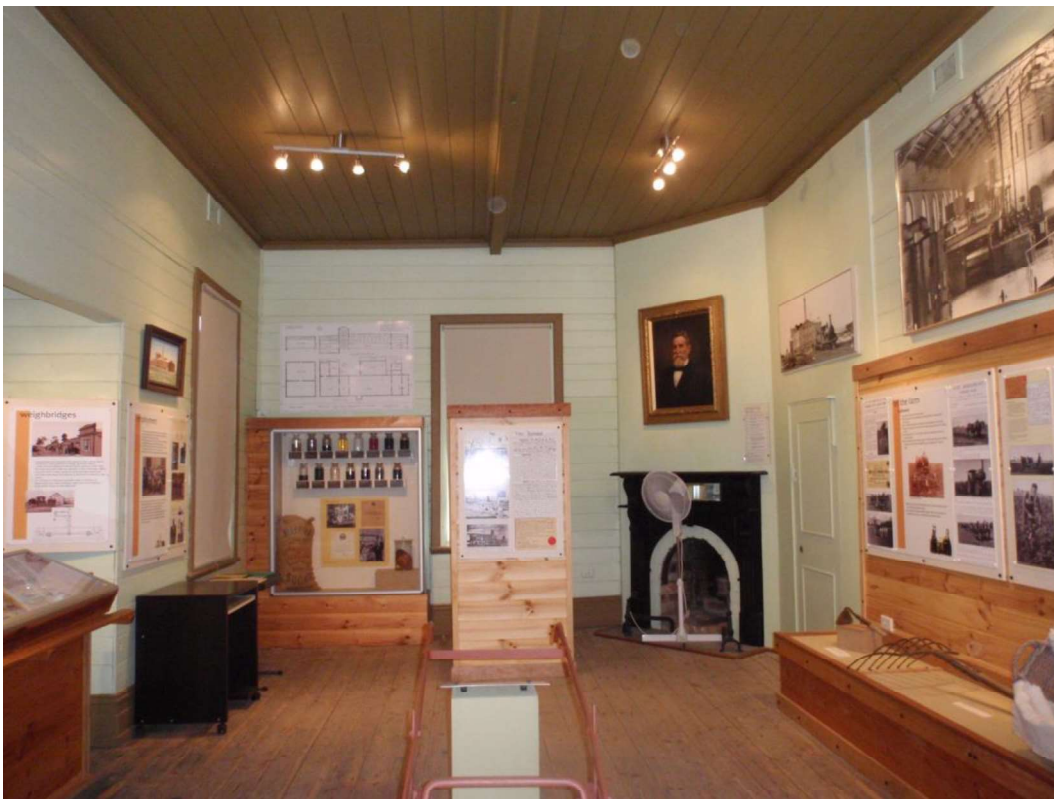
Figure D7. View of interior showing the timber lined ceiling, walls and floor, and the fireplace.
