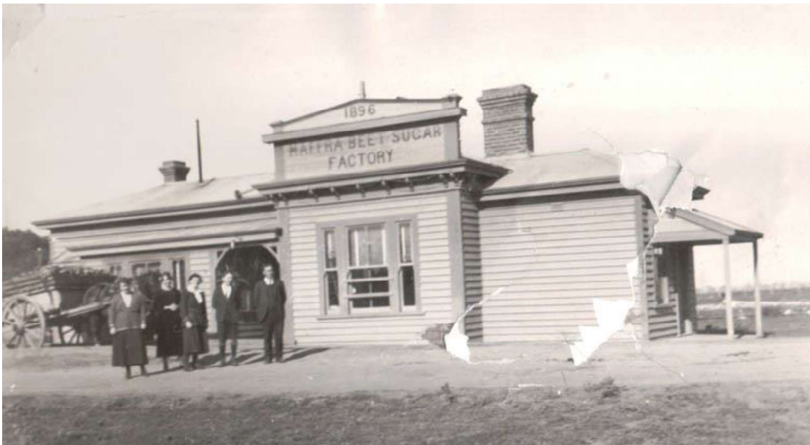
Figure H3. An early photo of the office (date not known), showing the verandah on the elevation to the right (since removed) and chimneys (MDHS, ID. P02174VMFF).
