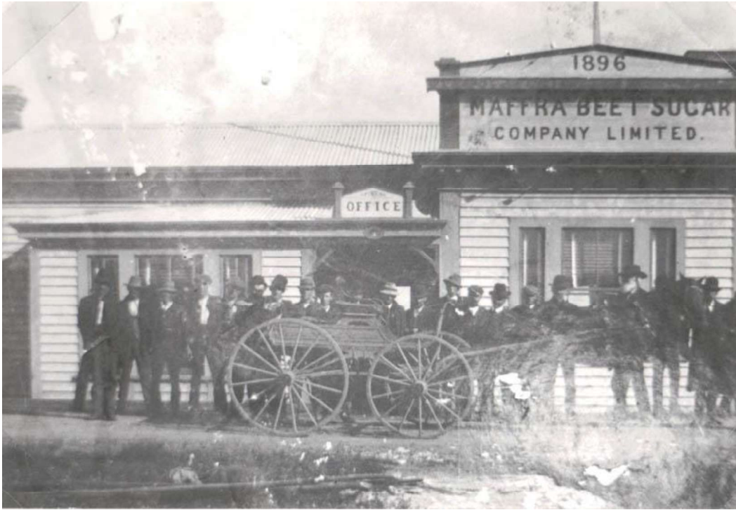
Figure H2. An early photo (date not known) of the office at its original location. The parapet reads 'Maffra Beet Sugar Company Limited' (MDHS, ID. P02172VMFF).
