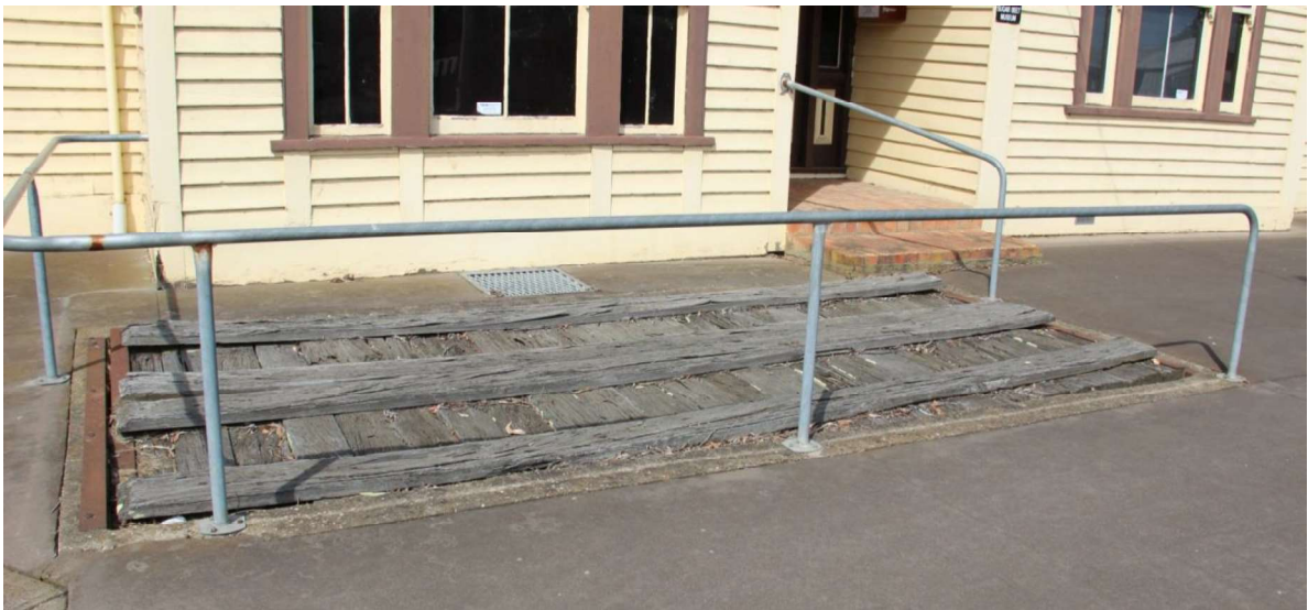
Figure D5. The original weighbridge as evident from above ground.
