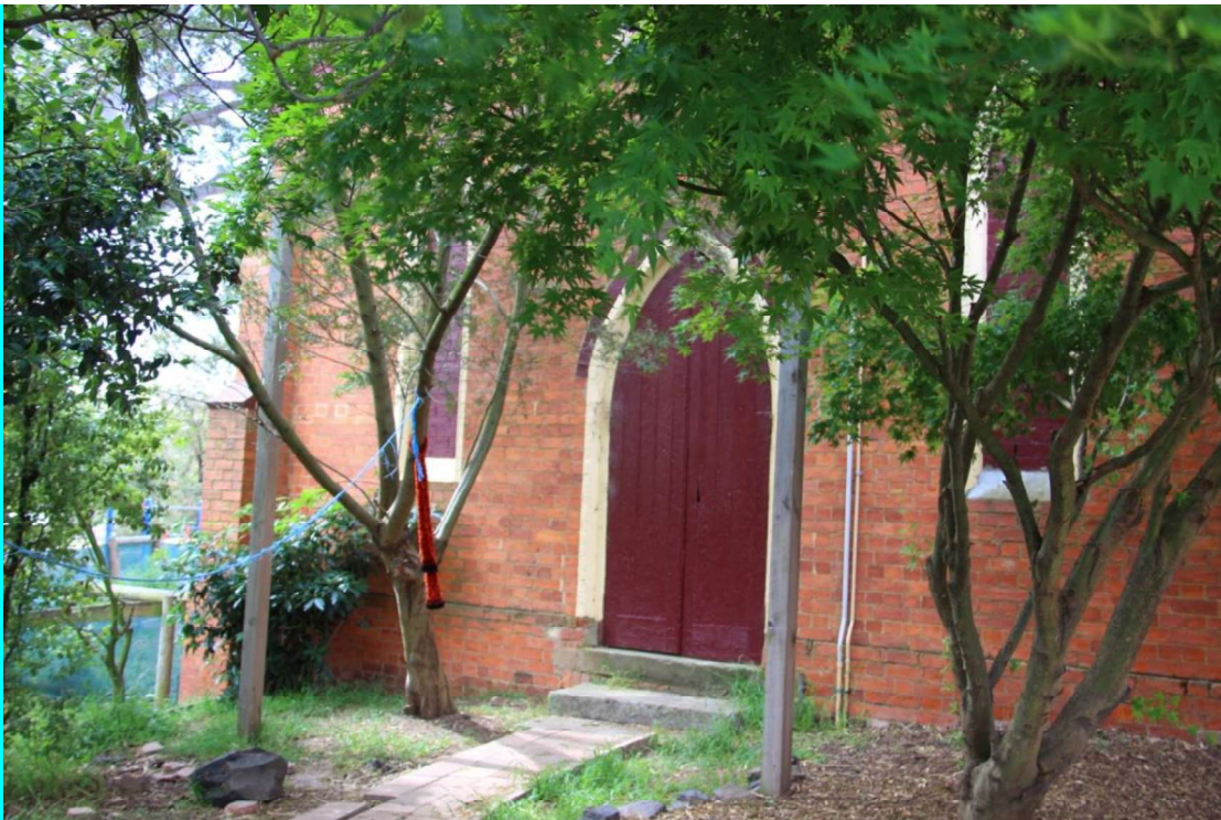
Figure D2. The facade (although difficult to see behind close foliage) has a central entrance with a pointed-arch and double timber ledged and framed doors, with a rendered surround (overpainted). The entrance is reached by two steps. To either side are two single pointed-arch
