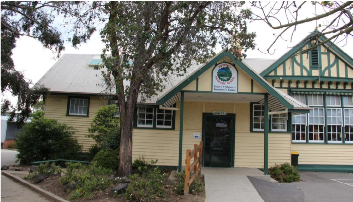
Figure D7. The facade facing Temple Street, comprises a large gabled-end to the right side and a central entrance. The central entrance is a wide opening that enters a projecting hipped-bay. Windows sit beneath the eaves of the bay, alternating with panels of roughcast render and timber strapping.
