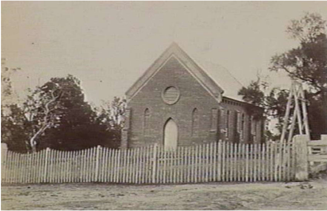
Figure H1. Early photos (date not confirmed; post-1886 when the fence was erected) showed the facade as it appears today, facing Harbeck Street. The east elevation formed three bays . A structure that is probably a bell tower was located to the west of the church (since removed) (HDHS).
