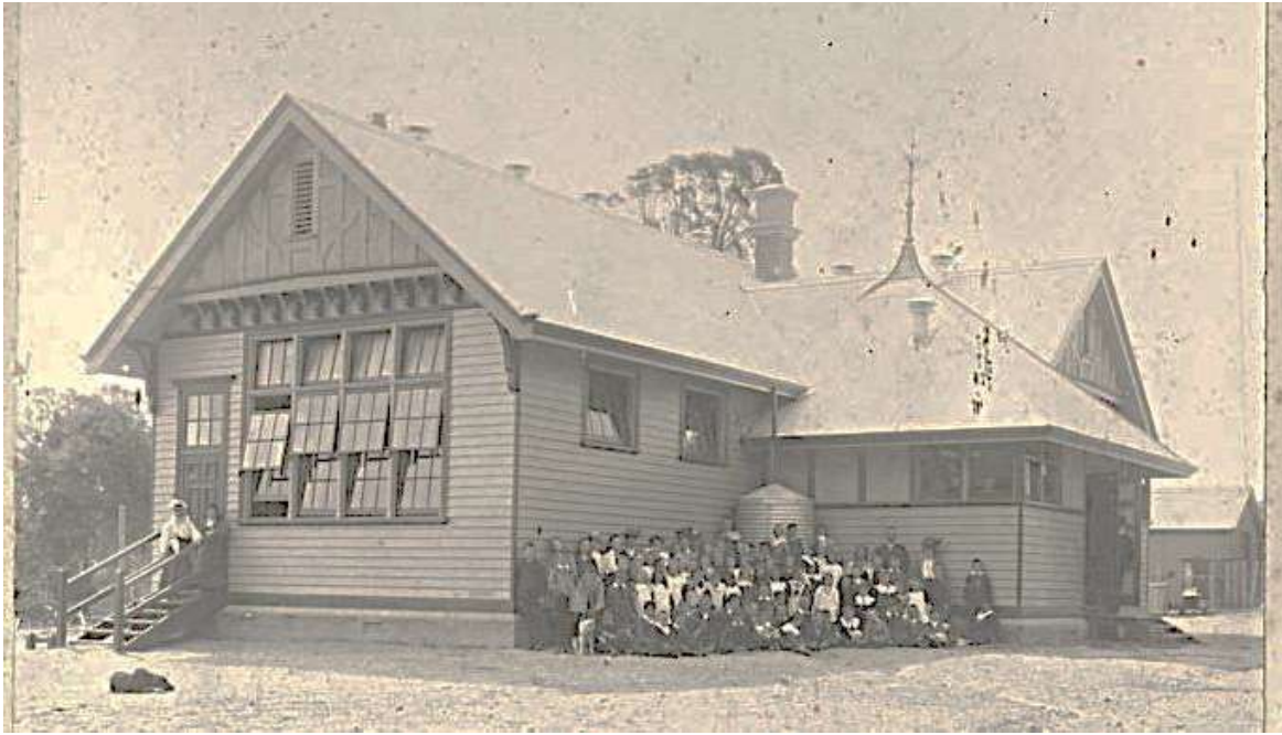
Figure H3. An early photo, before the addition of the western portion of the school building. The large southern elevation and its gabled-end appeared as it does in 2015, with an entrance left of the window bay, with highlights above (since covered over) and a timber staircase (since replaced). The east elevation had (left to right) two high windows, next to the hipped-roof bay (with a lower roofline) which had an ornate pinnacle at its peak (since removed) (HDHS).
