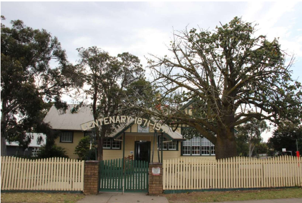
Figure D10. The entrance to the school on the east boundary is a gate with brick piers and metal gates (with attached palings). Above is a metal arch with letters reading 'Centenary 1871-1971', suggesting this entrance was built in 1971. Inside the boundary to the right of the entrance is a large Lacebark Tree ( Brachychiton discolor ).
