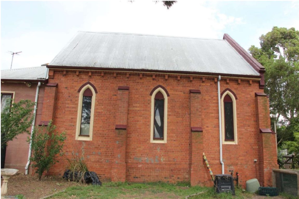
Figure D3. The west elevation. The side elevations comprise three bays, divided by four tall buttresses with rendered coping. Each bay has a single pointed-arch window with plain glass and a rendered surround (overpainted) and radiating (half) voussoirs (overpainted) at the arch. There are no sub floor vents.
