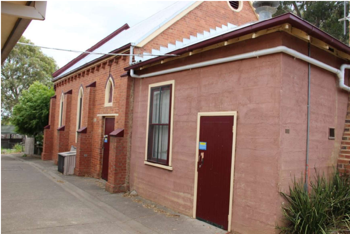
Figure D1. The east elevation. The modest church is constructed of red-brick in an English bond, with a brick plinth and gabled roof clad in (recent) corrugated iron and a rendered (overpainted) parapet to the facade (south elevation).
