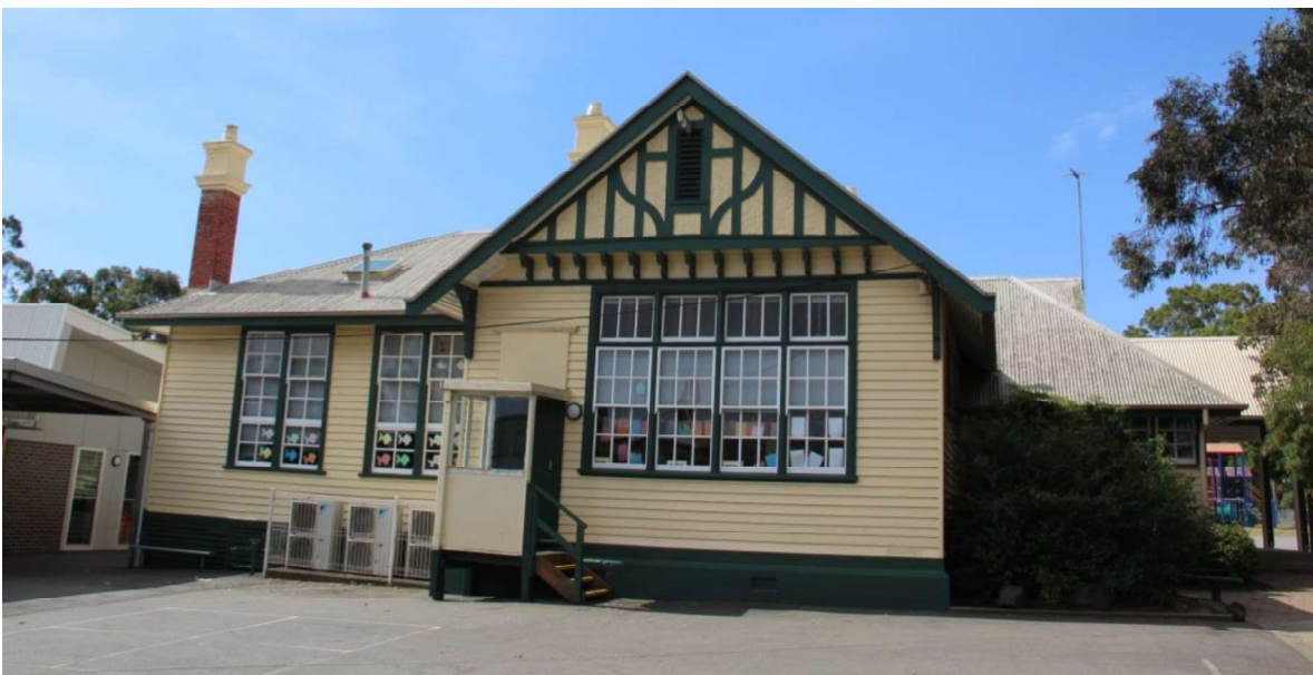
Figure D8. The south elevation (facing Harbeck Street) of the 1907 building has a large gabled bay. The western section of the building with a hipped roof was not constructed in 1907 (see Figure H3) but probably soon after, as it has the same architectural details and chimney as the 1907 building, however it does not sit on a masonry plinth.
