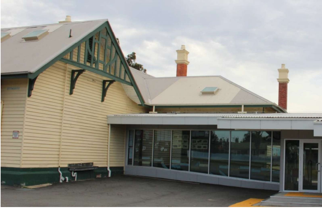
Figure D9. The west elevation has a large flying timber valance to the gabled-end, supported by timber brackets, with similar curvilinear details as the timber strapping of the other gables.
