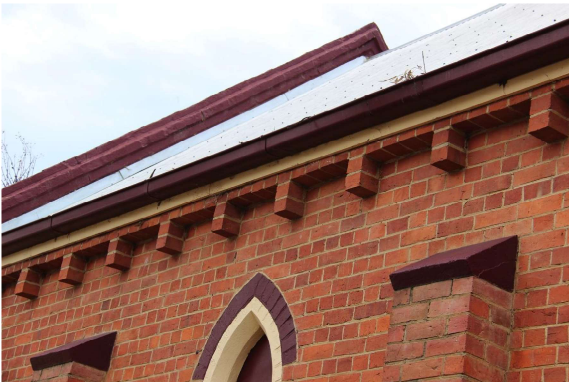
Figure D4. Architectural details: corbelled eaves decoration, rendered buttress coping, pointed
