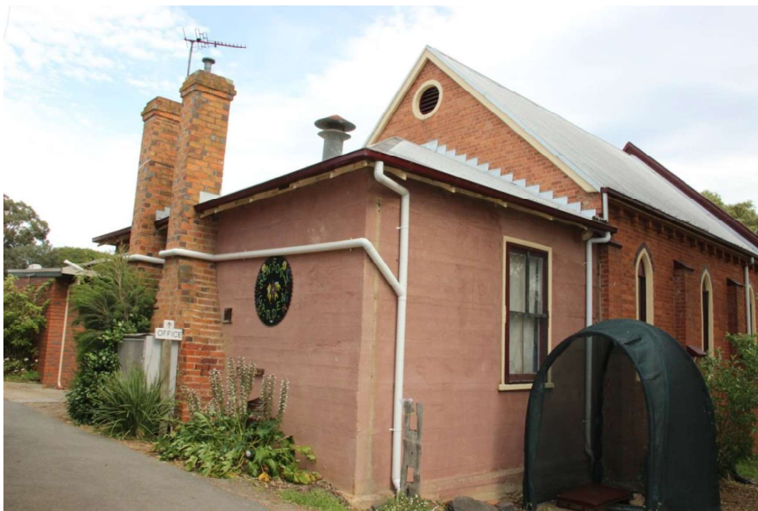
Figure D5. The north elevation of the 1875 church has a small round vent to the top of the gabled-end. To the rear (north) of the church is the concrete construction addition which is not significant. To the rear of this addition are two early large external brick chimney stacks with corbelled caps.
