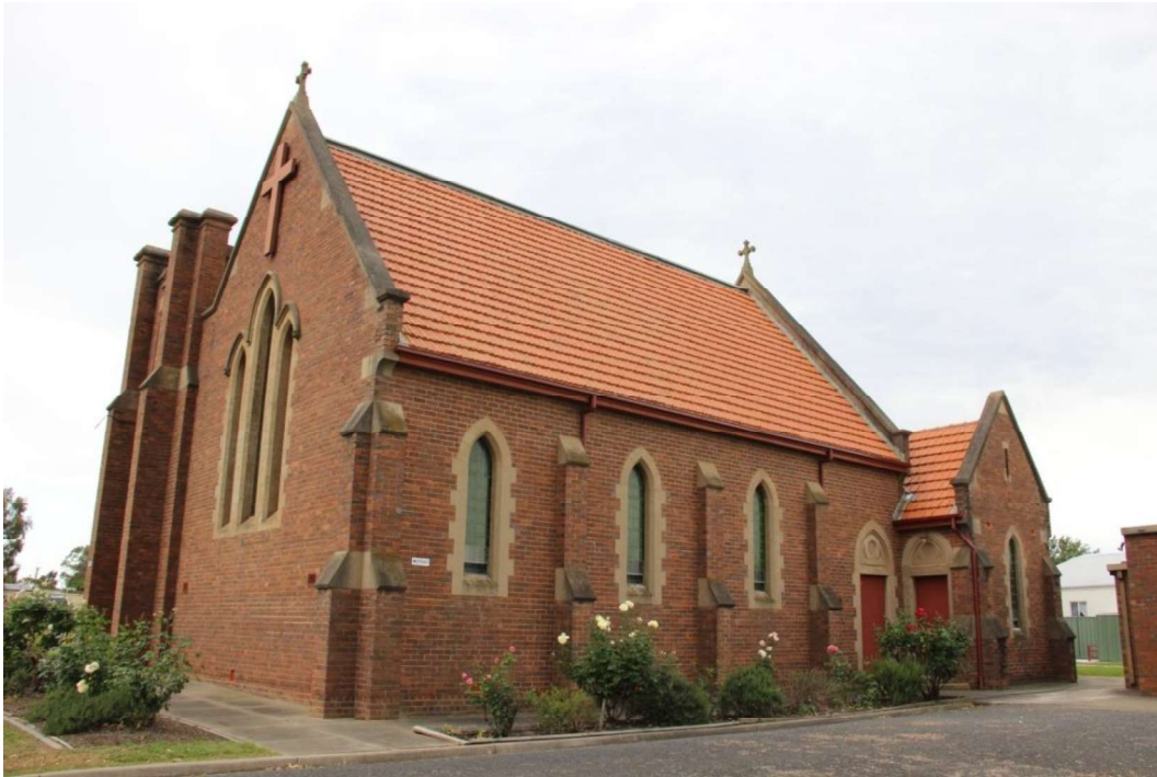
Figure D3. The south elevation. Timber ledged and framed doors on the side elevations and vestries have a bold pointed-arch pediment with a trefoil motif, surmounted by a label moulding stopped by rosettes. At the east end of the nave are vestries, which project to the north and south off the central chancel, which have the same treatment as the main portion of the church.
