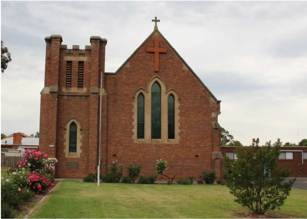
Figure D1. The substantial (handmade) red-brick church has a steeply-pitched gable roof that is hidden from Temple Street by a parapeted gable, with a cross at the peak of the gable. A dominant and tall castellated bell tower is located to the left of the facade.
