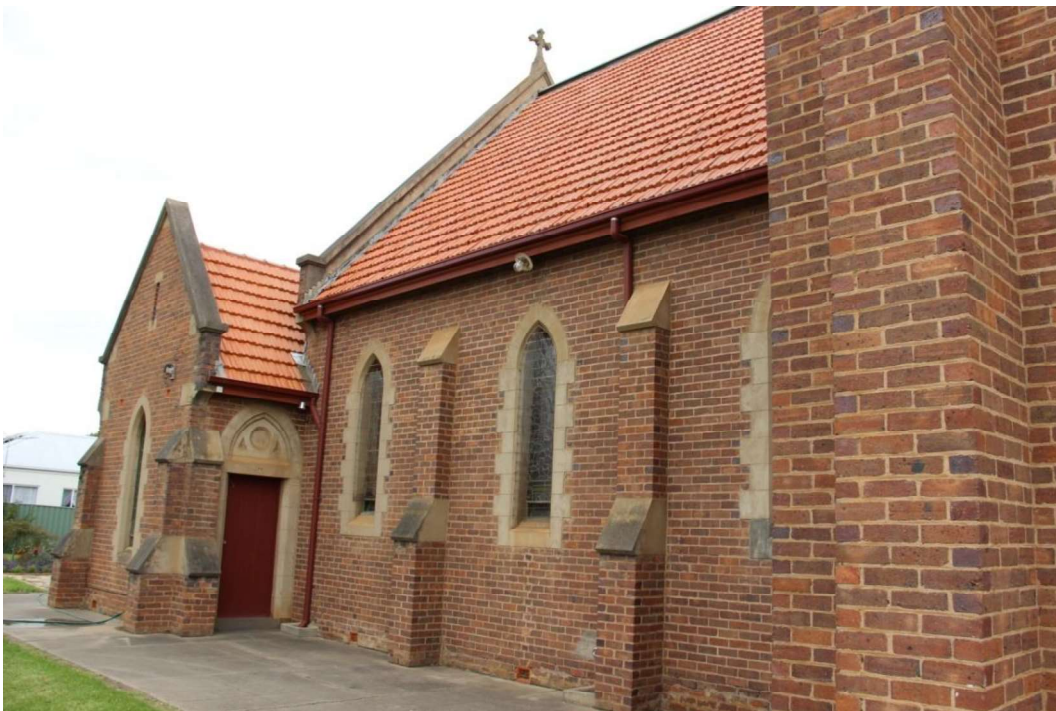
Figure D2. The north elevation. The gabled roof of the nave and eastern sections of the church are clad with terracotta tiles, as evident from the side elevations. The side elevations are broken into four bays by tall buttresses. Each bay consists of one pointed-arch window with quoining, and pictorial or geometric coloured leadlight. The north elevation contains two pictorial leadlight memorial windows towards the chancel end.
