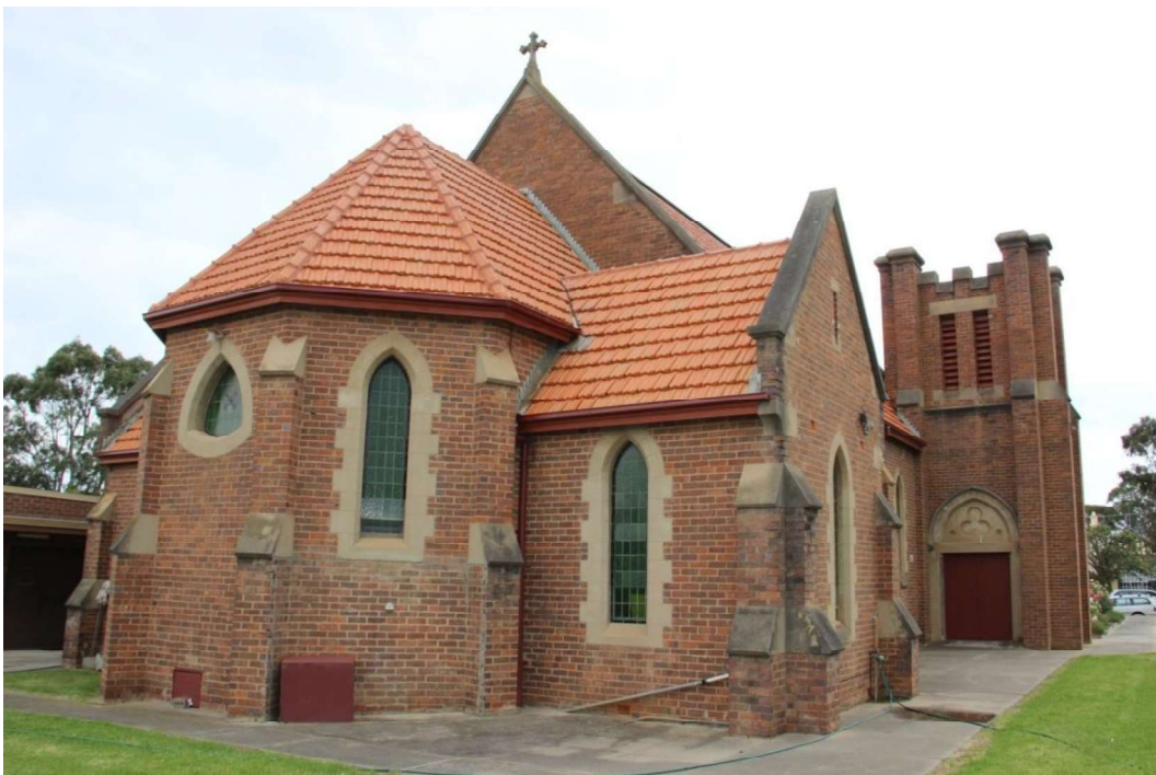
Figure D4. The east end of the church. The chancel is a faceted bay, also with the same treatment as the nave. Buttresses at the corners of the bay separate pointed-arch windows surrounded with quoining, with leadlight and a central small window in a triangular shape, with leadlight (with a floral motif).
