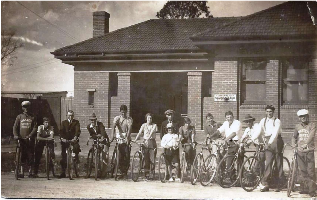
Figure H1. Photo of the post office taken c1927, soon after the post office was built, illustrating the original colour scheme of unpainted render and dark-tone timber joinery. (HDHS).
