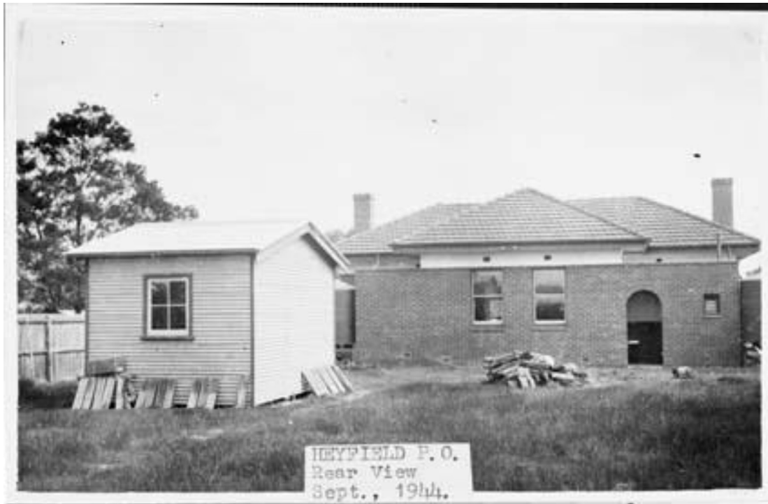
Figure H3. The rear elevation in 1944, with a round arched doorway and a small timber outbuilding to the rear of the post office (NAA).
