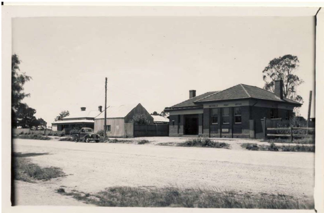
Figure H4. The facade and south elevation, photo dates to post-1948 (HDHS).
