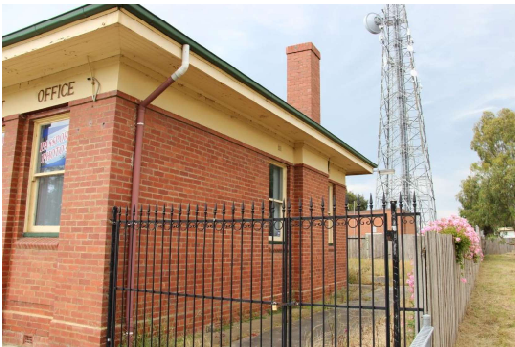
Figure D5. The southern elevation with the external chimney stack flanked by one-over-one sash windows.
