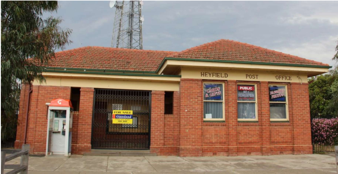
Figure D1. The façade of the post office. The two chimneys are out of view in this photo.
