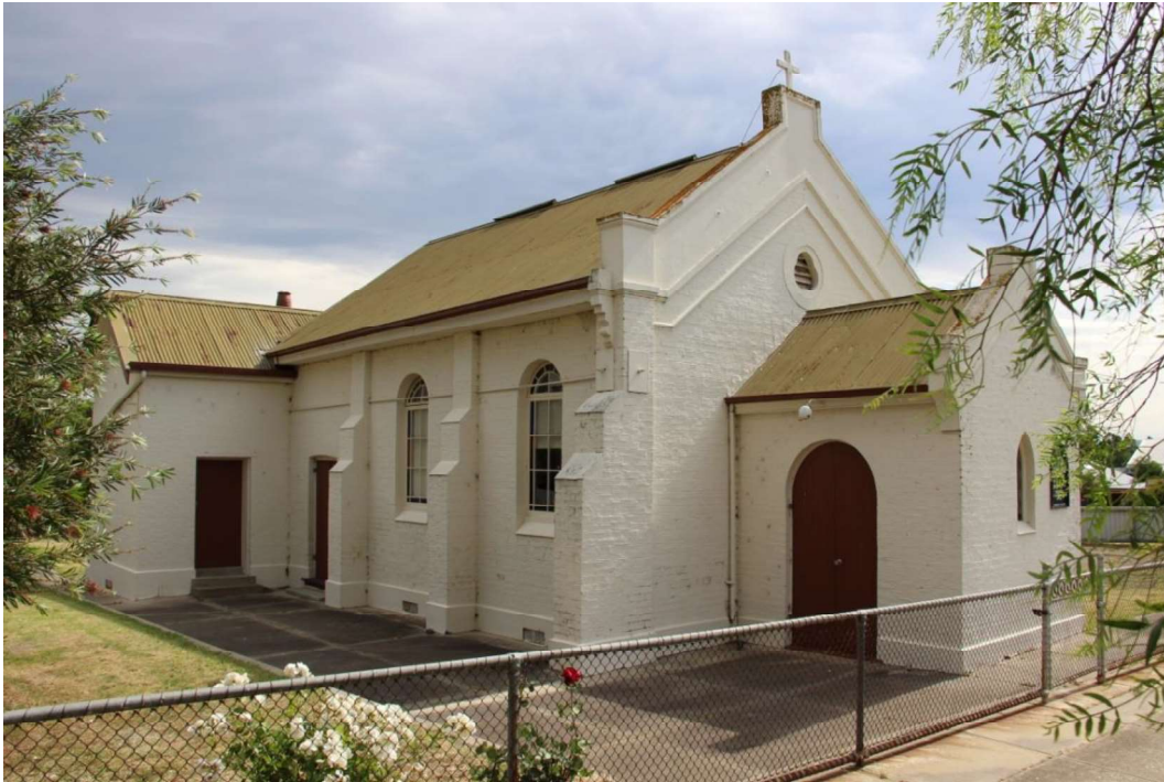
Figure D3. The east elevation. The vestry projects to the east off the vestry and is entered by a door facing north. Another timber door is located on the third bay of the east elevation. The entrance porch has a semi-circular arched door and opening on its east side.
