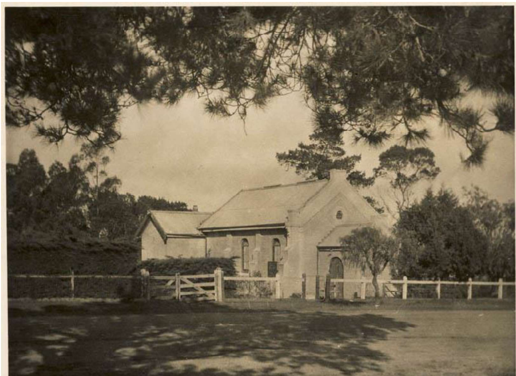
Figure H2. A photo dating post-1913, after the existing porch, vestry and buttresses to the side elevations were constructed (HDHS).
