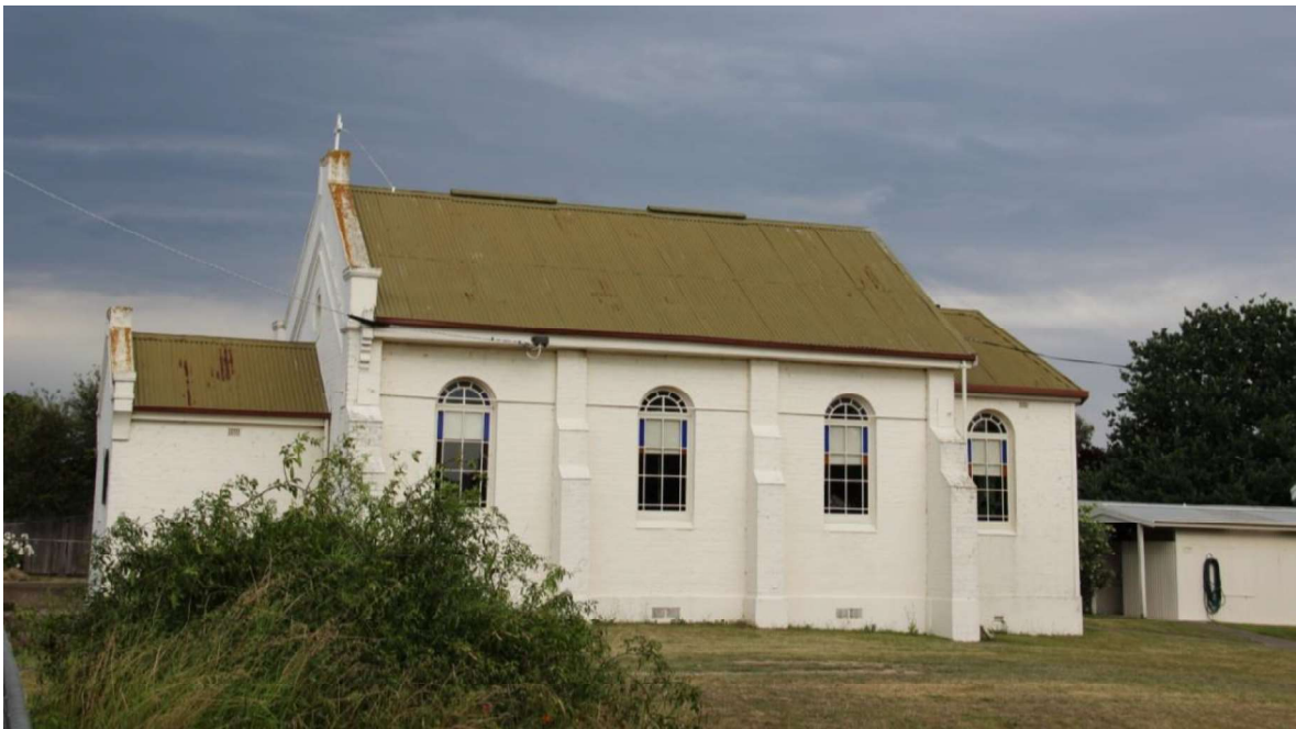
Figure D2. The west elevation. The side elevations comprise three bays created by buttresses (added in 1913). Each bay has a single semi-circular arched window. A chancel at the southern end of the church has a window of the same design on its west elevation.
