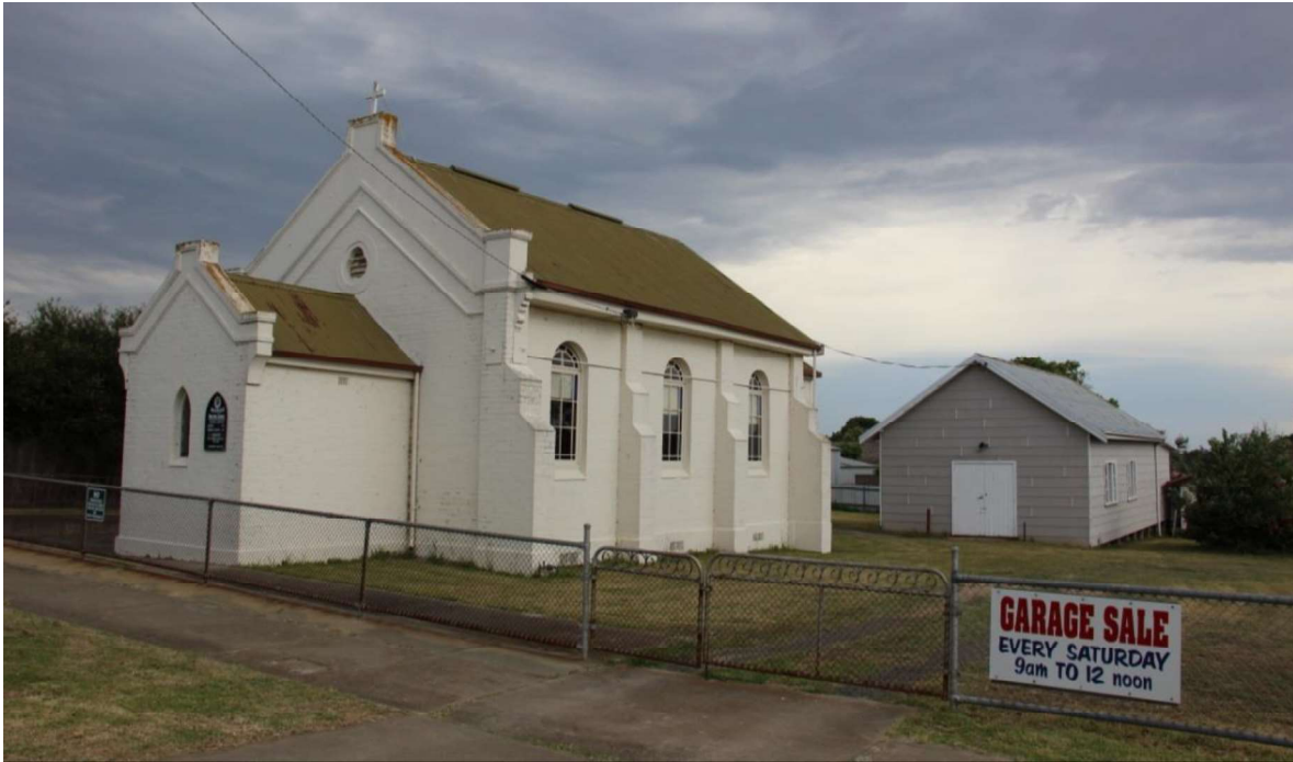
Figure D1. The brick (overpainted) church is modest in size and detail. The church has a gabled roof with a rendered (overpainted) parapeted gable to the facade. At the centre of the facade is a small entrance porch (1913), which imitates the details of the parapeted gable of the nave behind.
