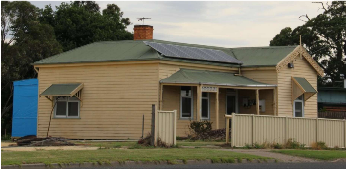
Figure D1. The facade and eastern elevation of the house. The weatherboard house has a shallow-pitched M-hip roof with a projecting gabled bay to the right of the façade, clad in corrugated iron. One red-brick chimney remains (one has been removed) and this has had the corbelled top section removed.
