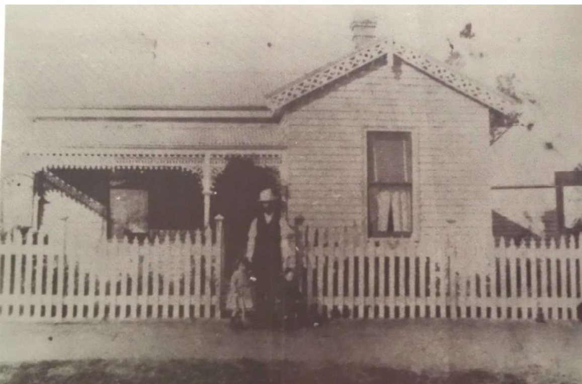
Figure H1. Constable Paddy Cox and a small girl in front of the police station in the 1890s. The facade at this date showed the roof clad with corrugated iron, corbelled brick chimneys (since removed or altered), the projecting gable bay with a decorative timber bargeboard and finial (the bargeboards remain in 2015; the finial has been replaced with similar) above a one-over-one sash window. The hipped verandah had a cast iron frieze in a timber frame and brackets. To the rear (right) of the house is a weatherboard outbuilding which was probably the original police stables (FitzGerald 1991:72).
