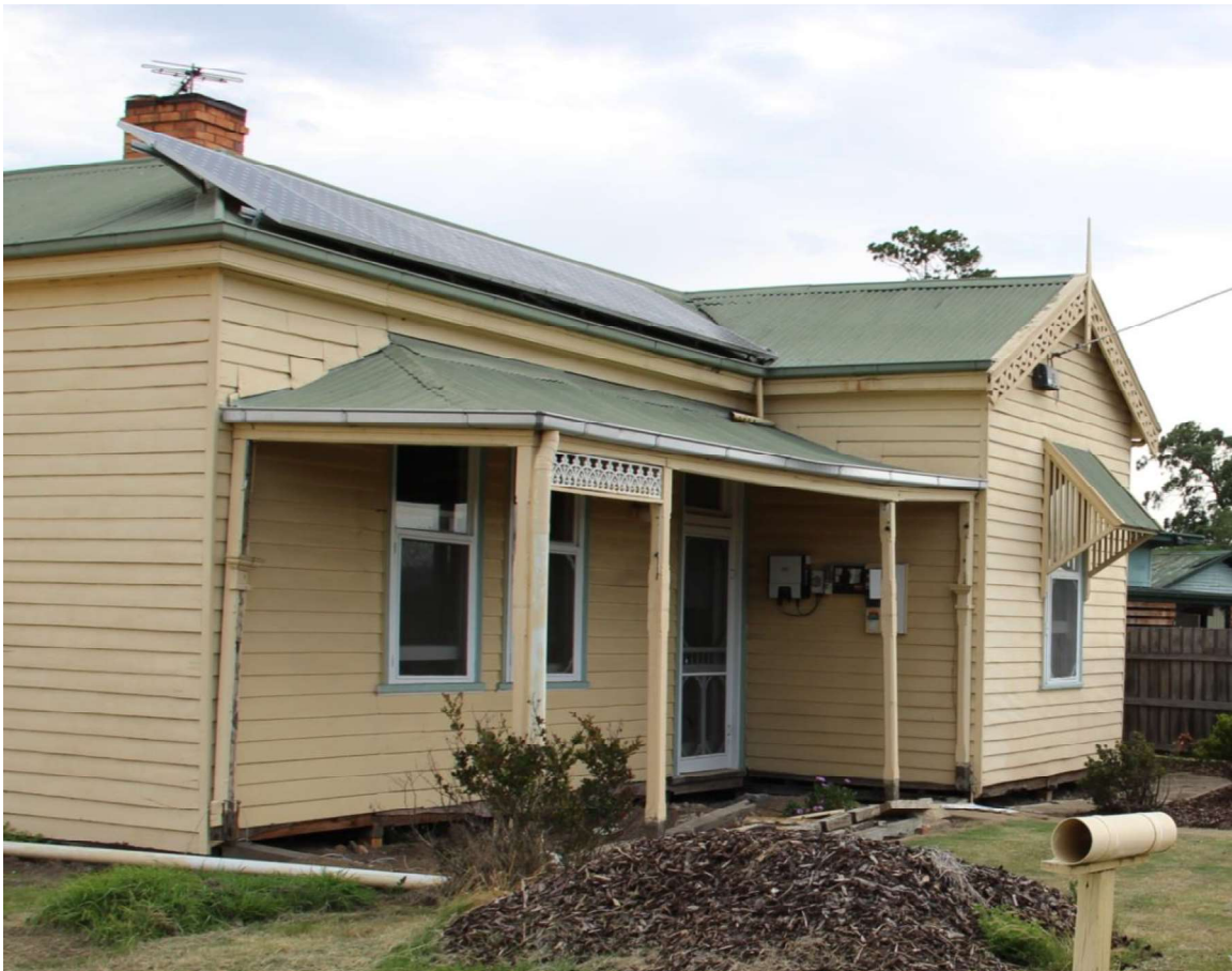
Figure D2. The facade with the projecting gabled bay to the right, with its decorative bargeboard and (not original) finial, and the hipped-roof verandah with most of the original cast iron removed. The remainder is located on the site below.
