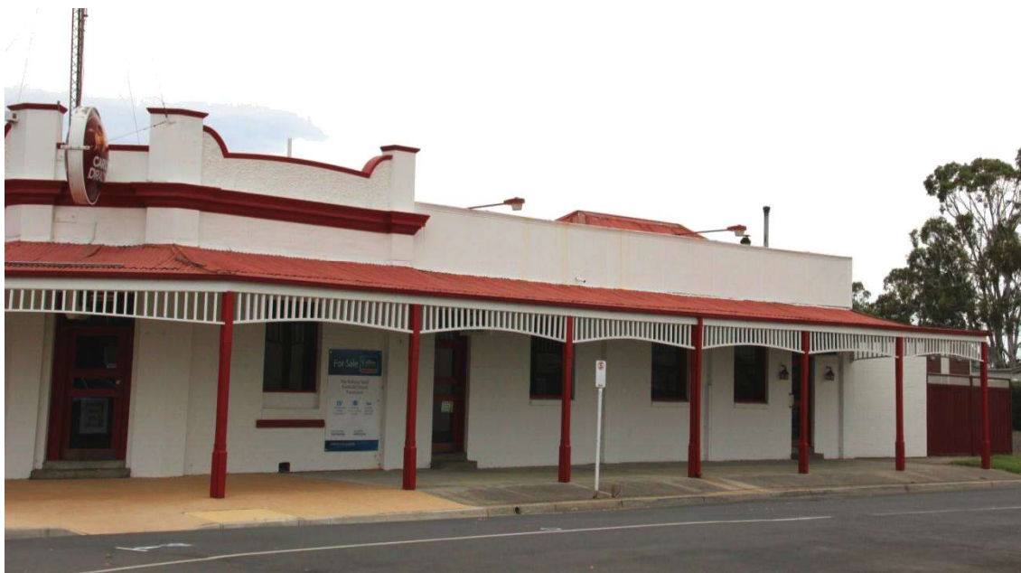
Figure D2. A shorter parapet constructed of simple panels is located at the south end of the west elevation (date not confirmed).
