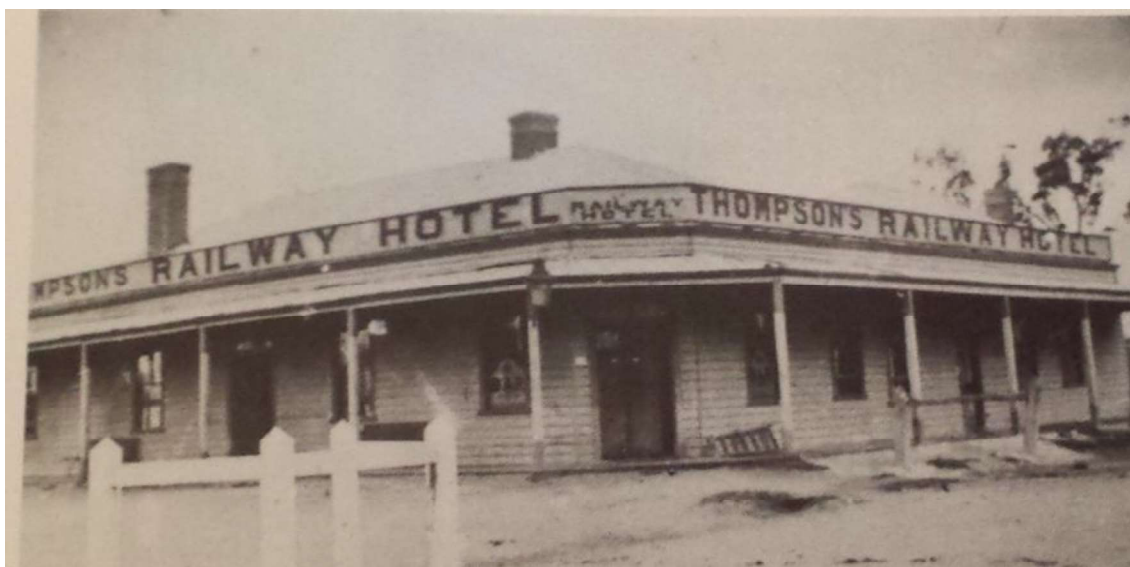
Figure H1. A photo dating to c1895 of the 'Thompson's Railway Hotel'. The photo shows the corner weatherboard building with a low parapet reading 'Thompson's Railway Hotel'. A hipped roof with two brick chimneys ran parallel to George Street, while a second hipped roof ran parallel with Pearson Street. A chamfered corner held the main entrance to the hotel, below a slightly concave skillion-roof verandah that continued along the two main elevations (FitzGerald 1991:21).
