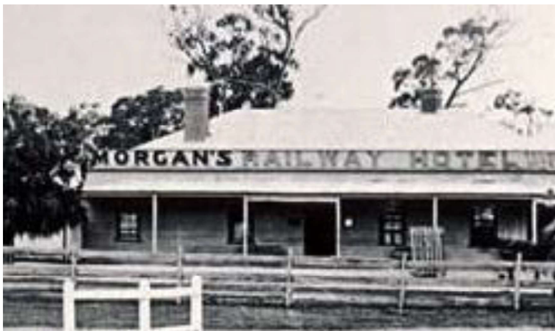
Figure H2. This photo dating to c1911 showed 'Morgan's Railway Hotel'. The hotel had a verandah, hipped roof and retained two brick chimneys (since removed) (HDHS).
