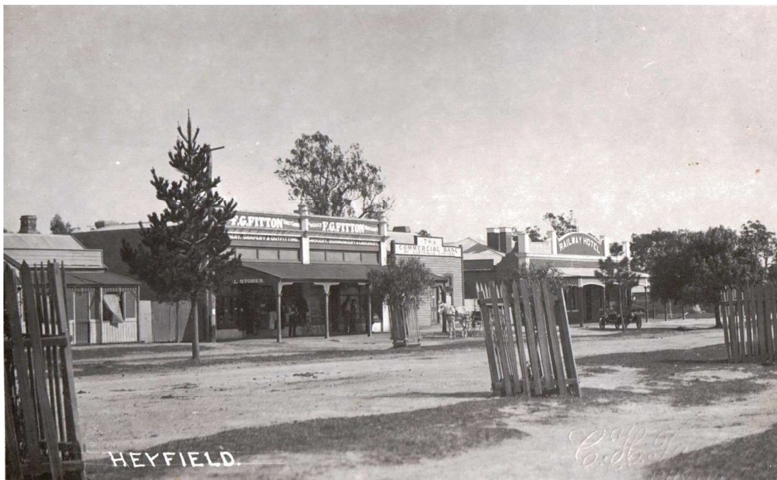
Figure H5. c. 1920s view of George St, Heyfield. Showing the George St elevation soon after it was constructed, was the same as in the 1975 photo in Figure H4. The tones of the colour scheme is also evident, such as the unpainted red brickwork, dark and light coloured rendered parapet, unpainted galvanised iron roof cladding, dark coloured verandah fascia and posts, and light coloured timber slatted verandah. It also shows the timber Commercial bank building owned by Bridget Clark.
