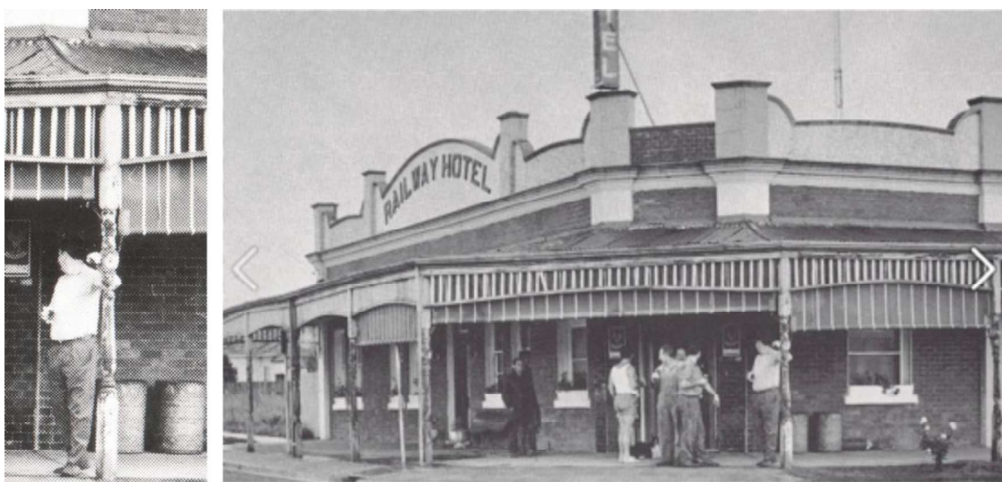
Figure H4. Photo showing the unpainted red brickwork, and the window and door fenestration which appears to match the Victorian era windows shown in Figures H1 and H2. The highly decorative turned timber posts and timber verandah valence are typical of the Federation era design ( see inset detail). Although this photo was taken in 1975 the building, including the verandah, as seen in this photo, is virtually unchanged from its appearance when it was built c1918.
