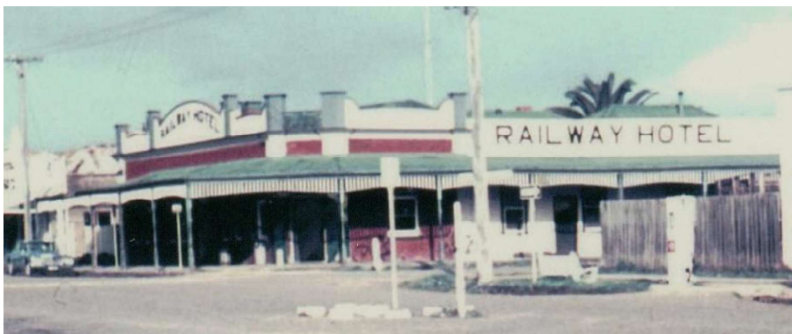
Figure H3. Photo dating to c1970s that shows the hotel with a timber parapet on the right hand side, and timber frieze (with vertical slats) running the length of the slightly concave skillion verandah at this date. The roof cladding was coloured green and 'Railway Hotel' was written on the shorted parapet fronting Pearson Street (HDHS).
