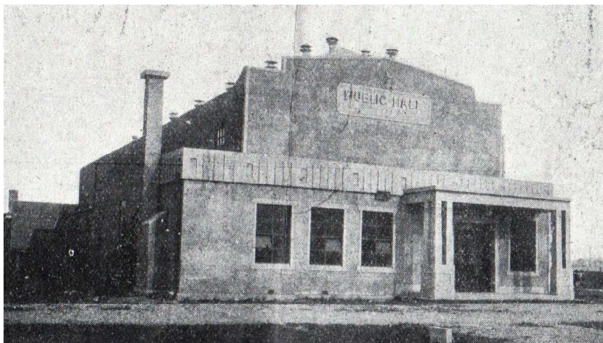
Figure H1. This photo showed the facade of the unpainted hall c1971, with many round vents to the roof (which have since been removed), the tall chimney on the east elevation and the entrance porch (Maddern 1971).
