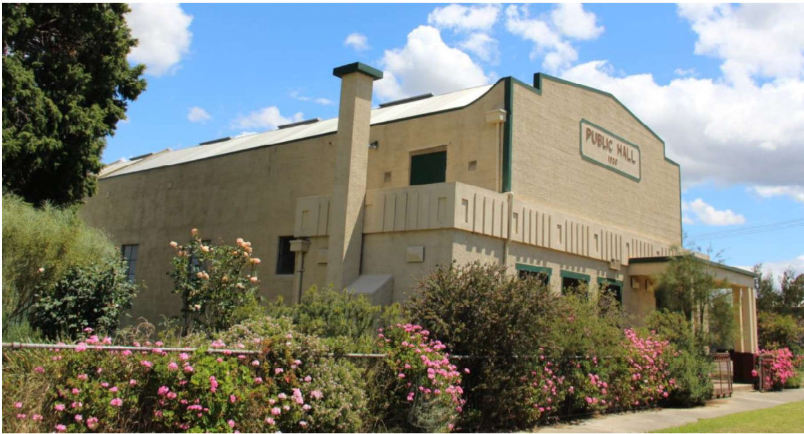
Figure D3. The height of the tall building is evident on the side elevations, which allows for a second floor behind the facade; with openings at this height and a balcony inside the hall. A tall rendered chimney with a simple flat cap is located on the exterior of the east end of the foyer.
