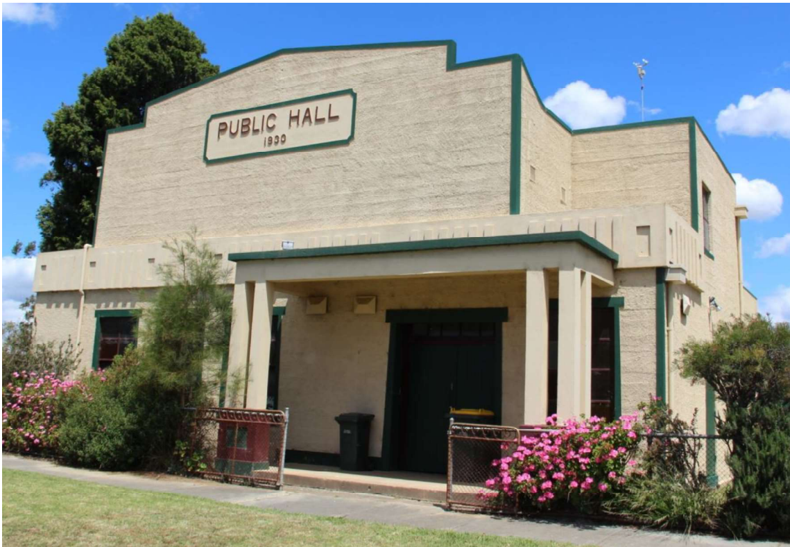
Figure D1. The hall sits behind a metal fence and gates which are likely to be original. The facade comprises a tall parapet that has a flat triangular pediment, and steps back at the sides. At the centre of the facade is a smooth-rendered panel with a rendered frame that reads 'PUBLIC HALL 1930' in relief. In front of the tall parapet is a wider section with a lower roofline, creating a foyer. Attached to the right is a flat-roofed entrance porch.
