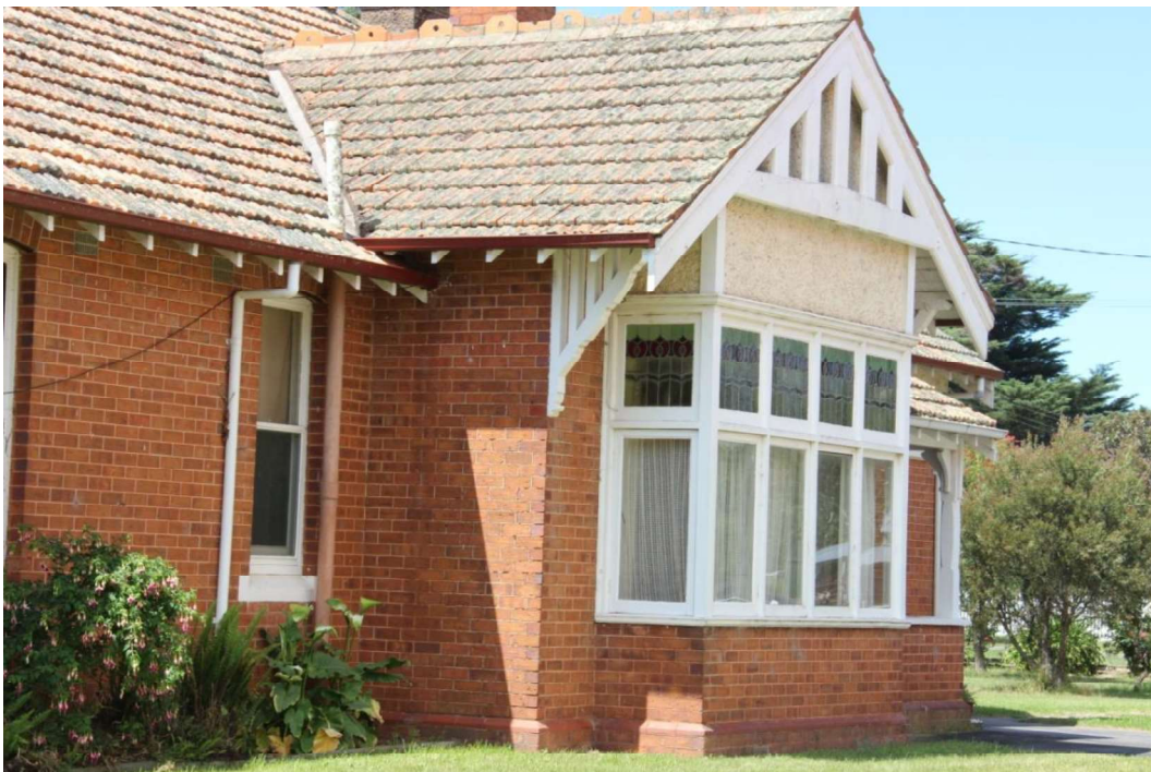
Figure D8. The gabled bay on the south elevation has a box window, with the top portion of the wall above the windows covered with rough-cast render, with a timber valance and large timber brackets to the gabled end.
