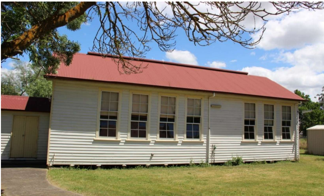
Figure D6. The north elevation of the hall has seven windows, each with a four-paned hopper (bottom) and four-paned sash window (at the top).
