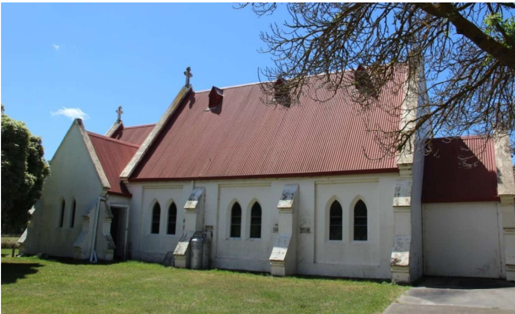
Figure D2. The side elevation of the church is divided into three bays by large buttresses. Above is the dominant roof with its dormer vents and to the rear (left) are the chancel and vestry.
