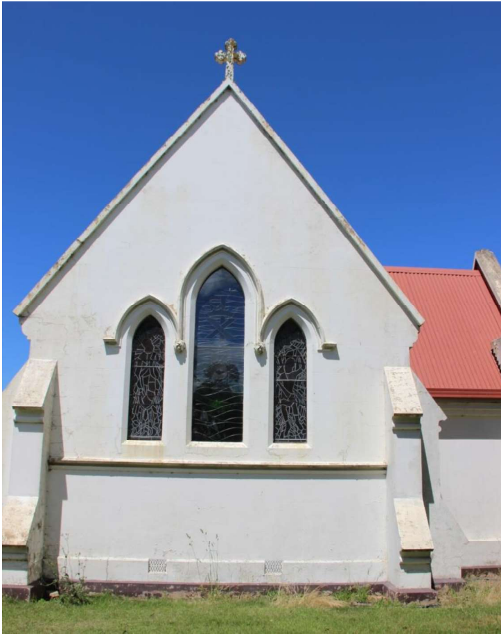
Figure D3. The west (rear) elevation of the chancel has three pointed-arch windows, with a label moulding stopped by rosettes. These three windows have pictorial leadlight.
