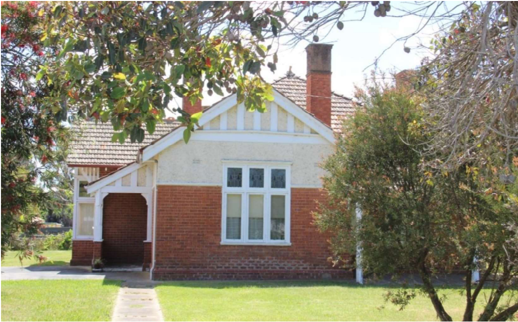
Figure D9. The façade has a gabled bay to Church Street, with rough-cast render and wide timber-strapping to the gabled end. The entrance is to the left of the gabled bay, under a porch created by the extension of the main roof.
