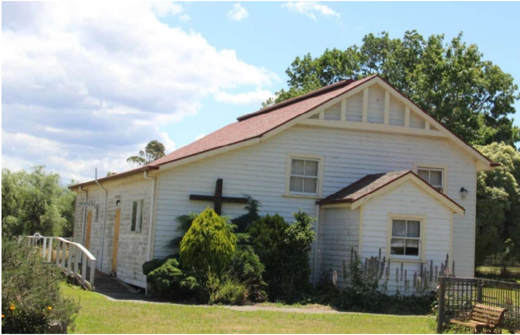
Figure D5. St Joseph's Hall is located to the south of the church and is a weatherboard building with a low-pitched gabled roof and a large skillion-roof addition off the south elevation which is not significant. A central entrance porch has a gabled-roof. The façade has small square two-over-two sash windows.
