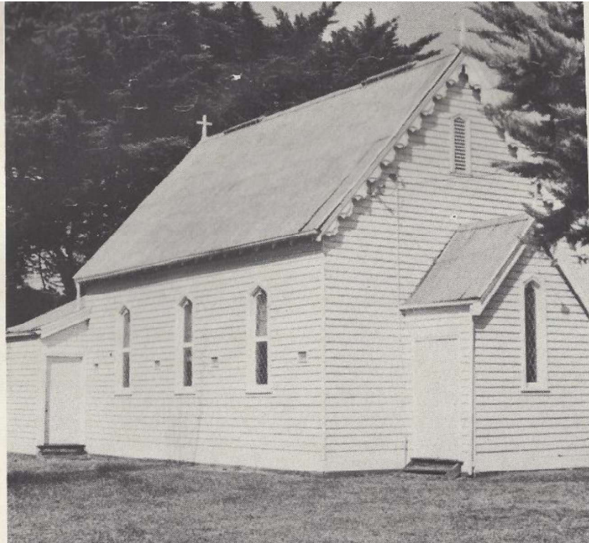
Figure H1. Photo dating to 1971 showing the gabled-roof timber building, ridge vents, Gothic leadlight windows, crosses at the gable peaks, entrance porch, and section to the rear. The large gable-end had a decorative bargeboard (which has since been removed) (Maddern 1971). This photo is evidence that the building remains very intact in 2016.
