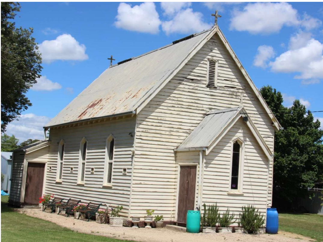
Figure D1. The facade of the church with the central entrance porch, with Gothic arched windows, a Gothic arched vent in the gable end and three crosses at the apex of each gable.
