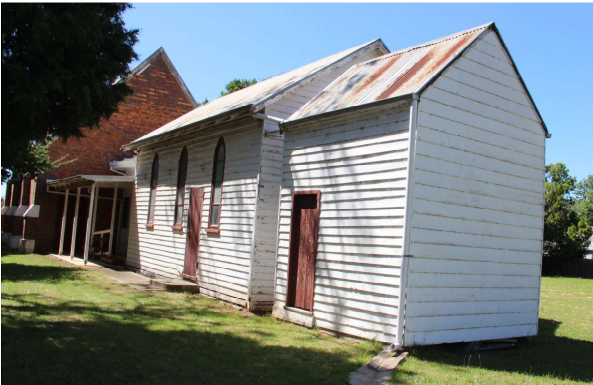
Figure D8. The north elevations of the weatherboard buildings to the rear of the 1908 brick church.
