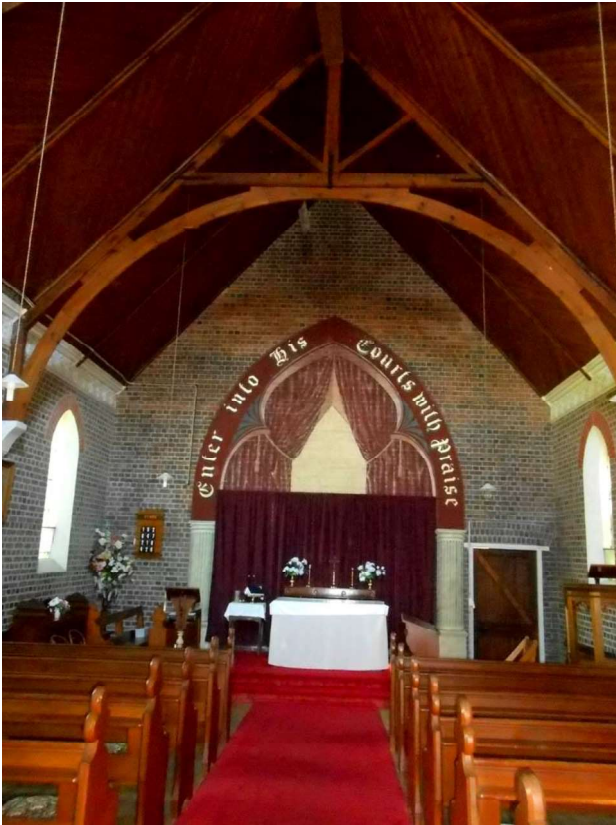
Figure D5. The interior of the church with its tuck pointed face-brick walls, decorative cornices and exposed timber roof trusses (MDHS).
