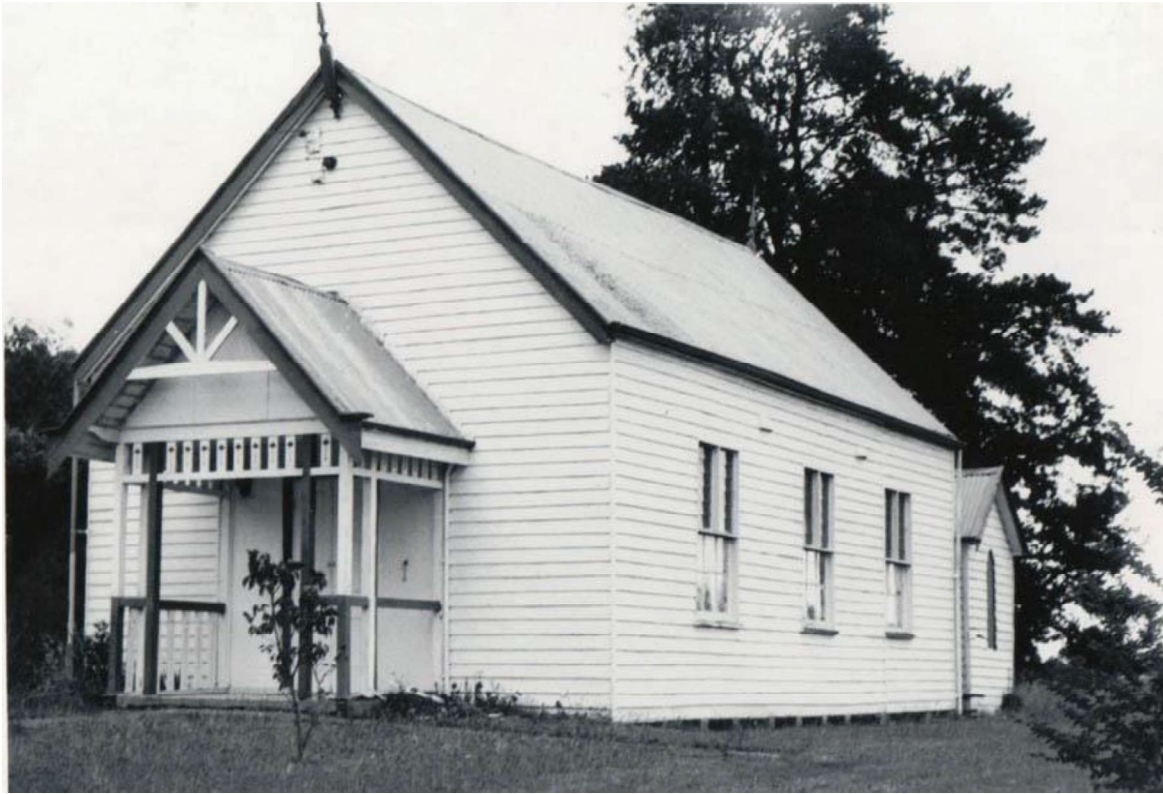
Figure H1. The church in 1976. The original porch with a pointed arch window had been relocated to the rear, and a c1970s porch added at the front. The top sashes of the side windows have been replaced with louvres. The finials to the roof evident here, have since been removed. (MDHS, ID. P02788VMFF 1976).
