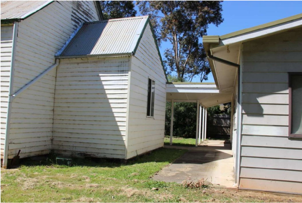
Figure D4. At the rear (west end) of the church is a small timber addition with a (uneven) gabled roof. To the west of the church is a modern weatherboard building.
