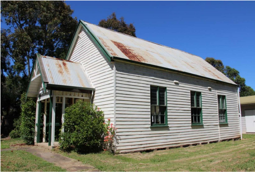
Figure D2. The modest weatherboard church has a gabled roof clad in corrugated iron, with simple bargeboards to the gabled ends, reflecting a simplified version of a Carpenter Gothic church. The side elevations consist of three windows, with six-paned sash windows to the bottom half, with a pair of modern louvered windows above.
