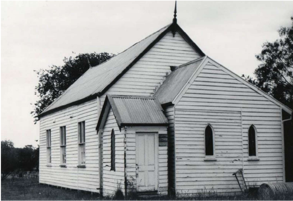
Figure H3. The rear elevation in 1975, showing the ‘relocated original front porch’ on the left (since removed), and an early addition to the right with similar pointed-arch windows (MDHS, ID P02785VMFF 1976).
