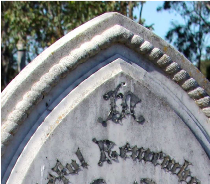
Figure D2. Detail showing the carved 'rope', gothic pointed arch, and deteriorating lead lettering on the marble memorial headstone.
