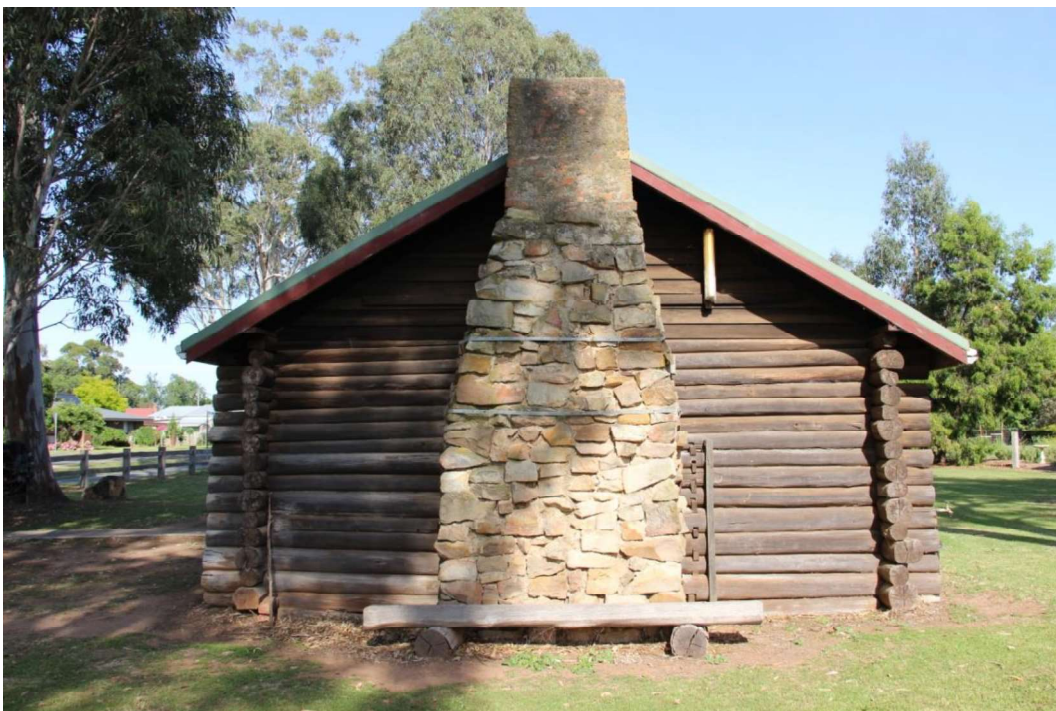
Figure D2. The east elevation with the large stone chimney stack, with a red brick top.
