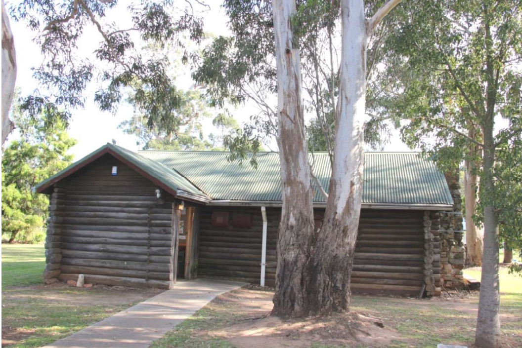
Figure D1. The south elevation of the cabin, which faces Avon Street. The entrance is off the east side of the entrance porch, to the left of the building.
