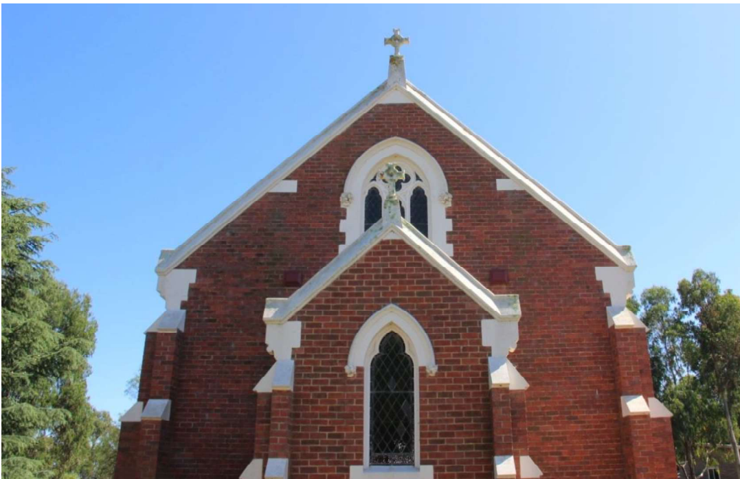
Figure D2. The church has pointed-arch window openings with a label moulding stopped by rosettes and a rendered sill. Recessed within each opening is a leadlight window (of coloured glass in a diaper pattern) which finishes at the top in a trefoil motif.
