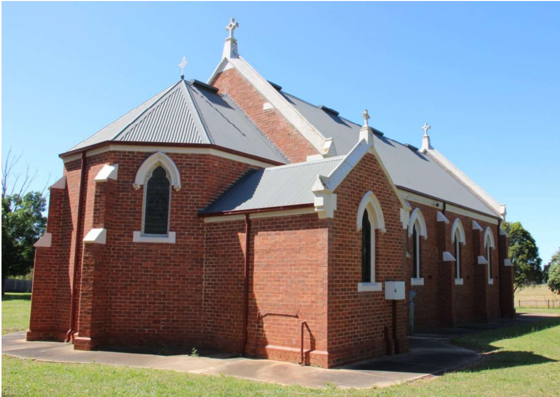
Figure D3. The side elevations form four bays, divided by five buttresses (all with rendered coping). At the (rear) chancel end of the church is a faceted bay with smaller windows at a raised height. Projecting off the west of this is a small vestry with a gabled roof.
