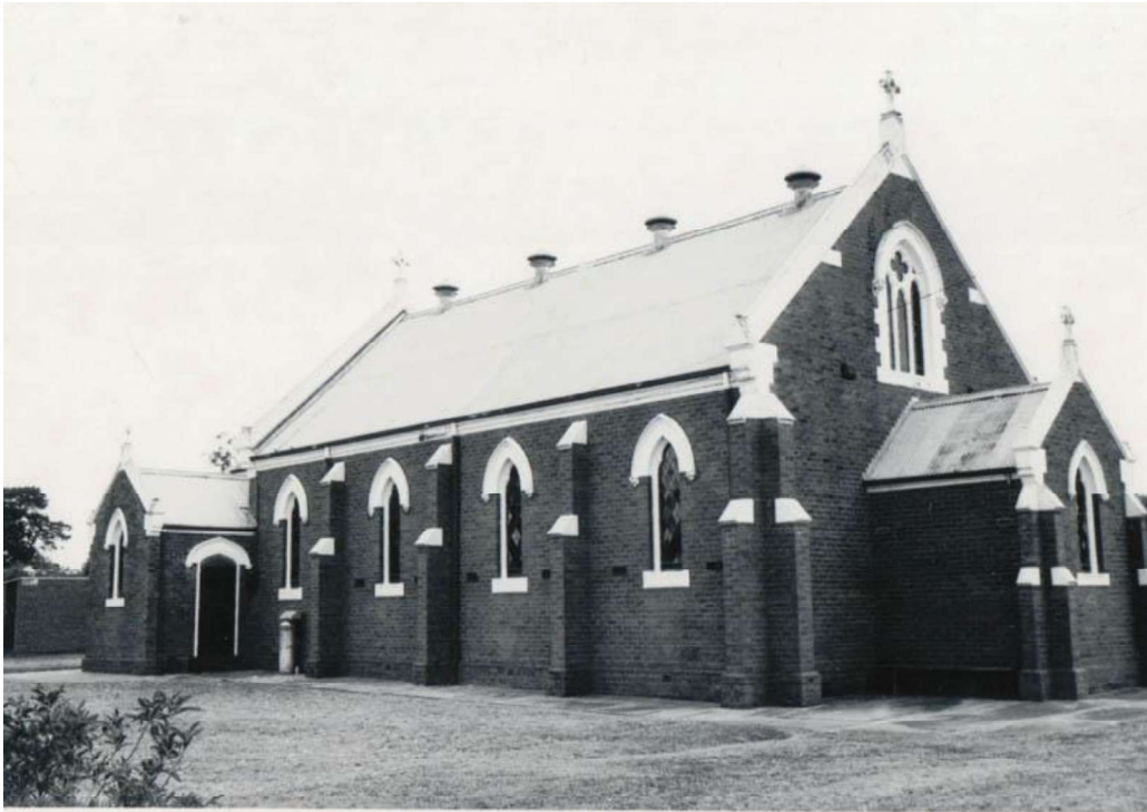
Figure H2. Photo dating to 1976, showed the vents along the ridge of the roof remained at this date and the rendered decoration had been overpainted (MDHS, ID. P02790VMFF 1976).
