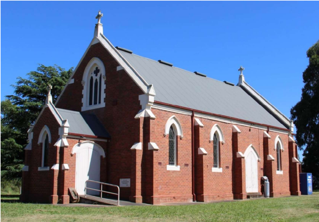
Figure D1. The church constructed of handmade red bricks, with its gabled roof and central entrance porch. Decorative render and coping is a decorative element of the Federation Gothic design, overemphasised by the recent white paint.
