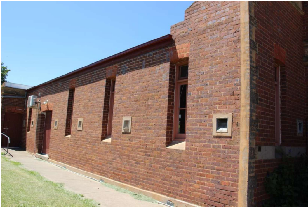
Figure D5. The north elevation with the double doors to the north elevation, and the single doors which enter the rear section of the 1904 building.
