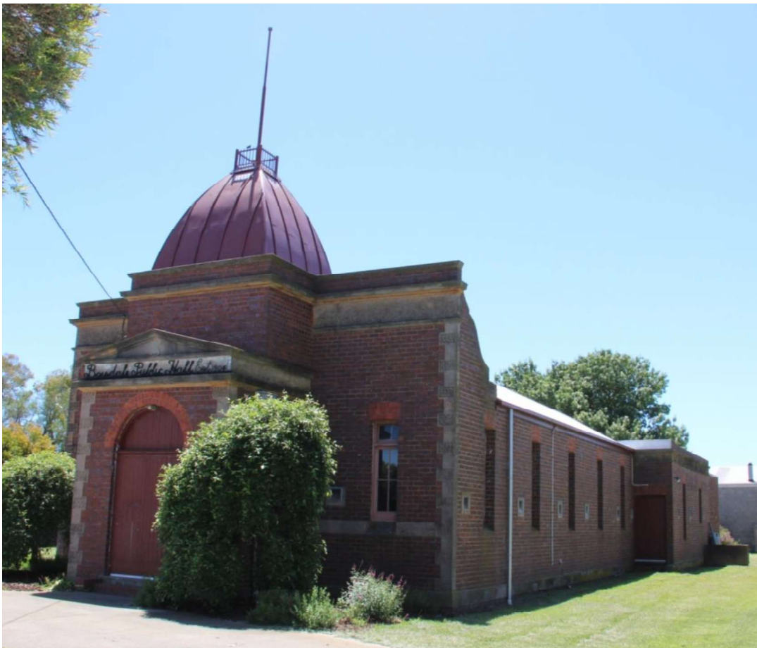
Figure D2. The brick hall with its dominating square dome with iron cresting and a flagpole, set behind the parapet. The building has red brick and smooth and roughcast rendered dressings.
