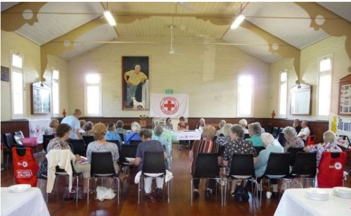
Figure D6. The interior of the hall, recently painted, showing the coved timber lined ceiling and decorative trusses. The World War I and II Honour Boards remain (MDHS, Helen Montague).
