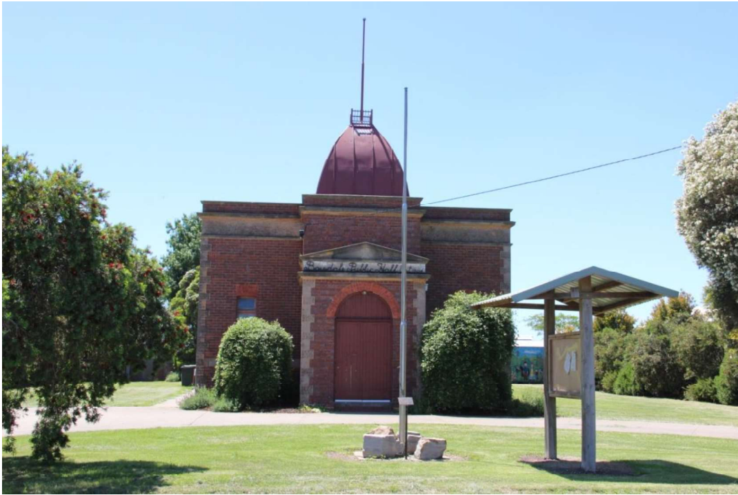
Figure D1. The hall setback in the lawn setting, reached by the circular driveway, with the flagpole on the front lawn. The town information board is outside of the title boundary, on the road reserve.
