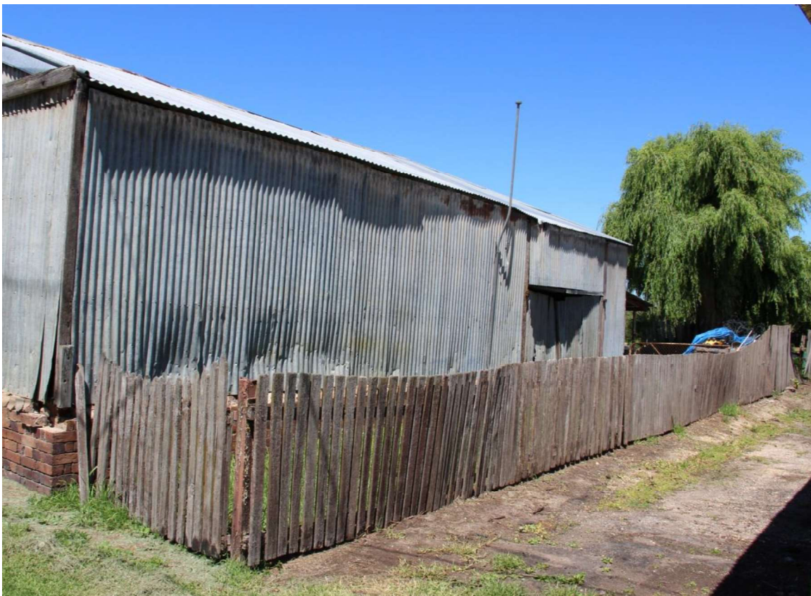
Figure D4. The north elevation of the blacksmiths and wheelwrights with one large opening near the rear of the building and a skillion-roof verandah off the rear elevation. The timber picket fence appears to be an early construction and may have been relocated to this location post-c1980.
