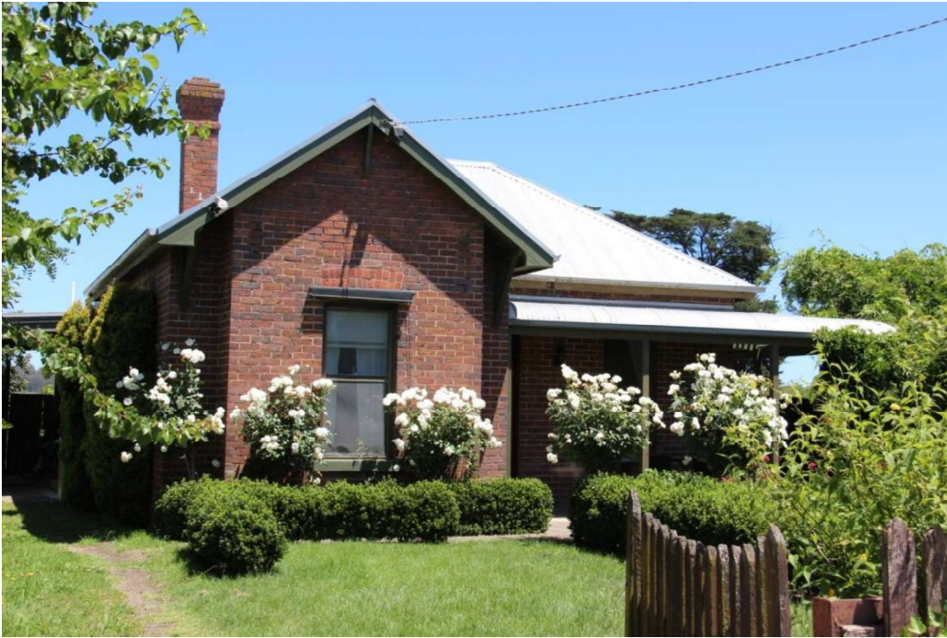
Figure D5. The blacksmith's house is a typical Federation era brick construction with a hip-and-gabled roof and projecting gabled bay to the left of the facade, and (modern) return verandah to the right. It is located in a garden setting with an early (possibly original) timber picket fence.
