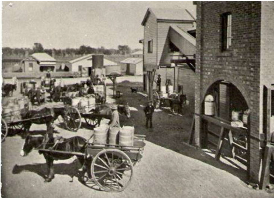
Figure H1. The Boisdale Cheese and Butter Factory and horse-drawn milk carts in the foreground, with the stables with skylights, blacksmiths and blacksmith's house in the background. Photo dates to c1910 (Boisdale Stables Project).
