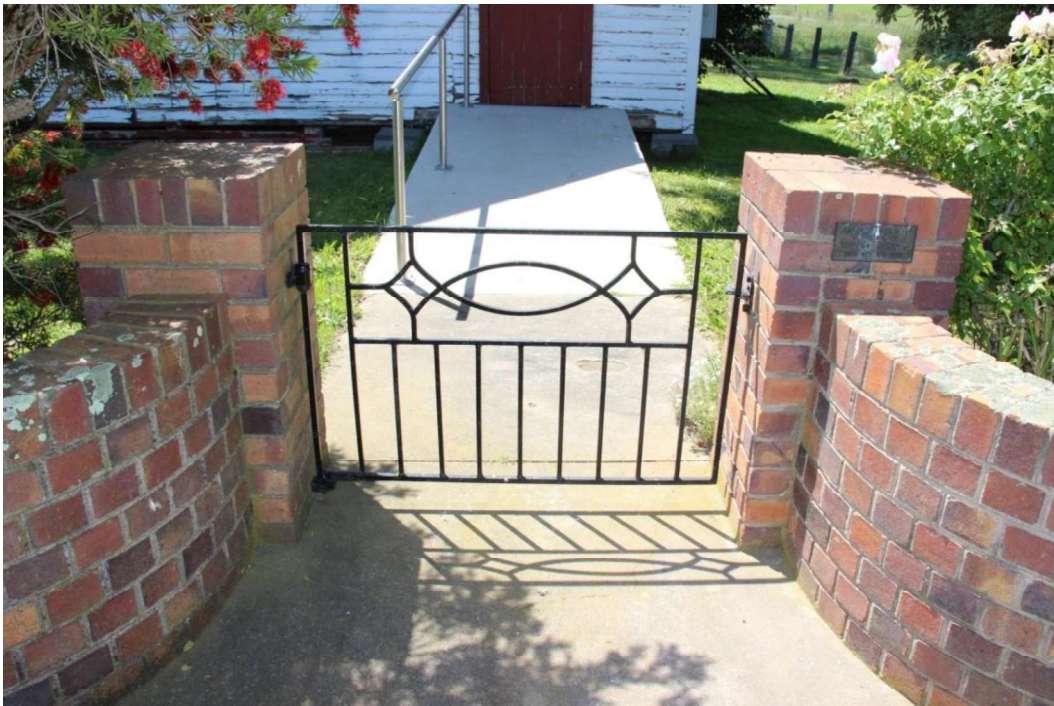
Figure D6. A 1950s brick fence and mild steel vehicular and pedestrian gates remain along the front (east) boundary. The brass plaque on the pier to the right of the gate states that it was erected in memory of Trevor Harvey, who died on 9 December 1952.
