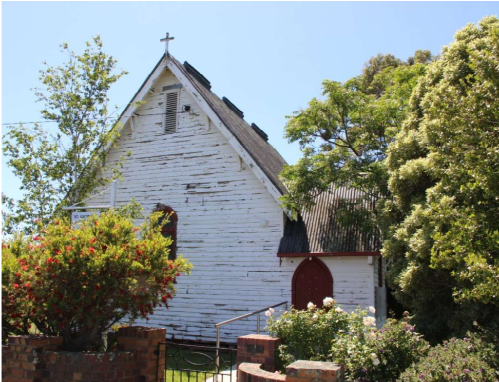
Figure D2. The entrance porch on the south elevation has a timber door with a pointed-arch on the west elevation. To the left is the Silver Birch ( Betula pendula ) first planted in 1967 was in memory of Mrs Ollie Clarkson. To the right is the White Cedar tree ( Melia azedarach ) and its associated plaque that commemorates the life of Gladys Tatterson (1899 – 1995).
