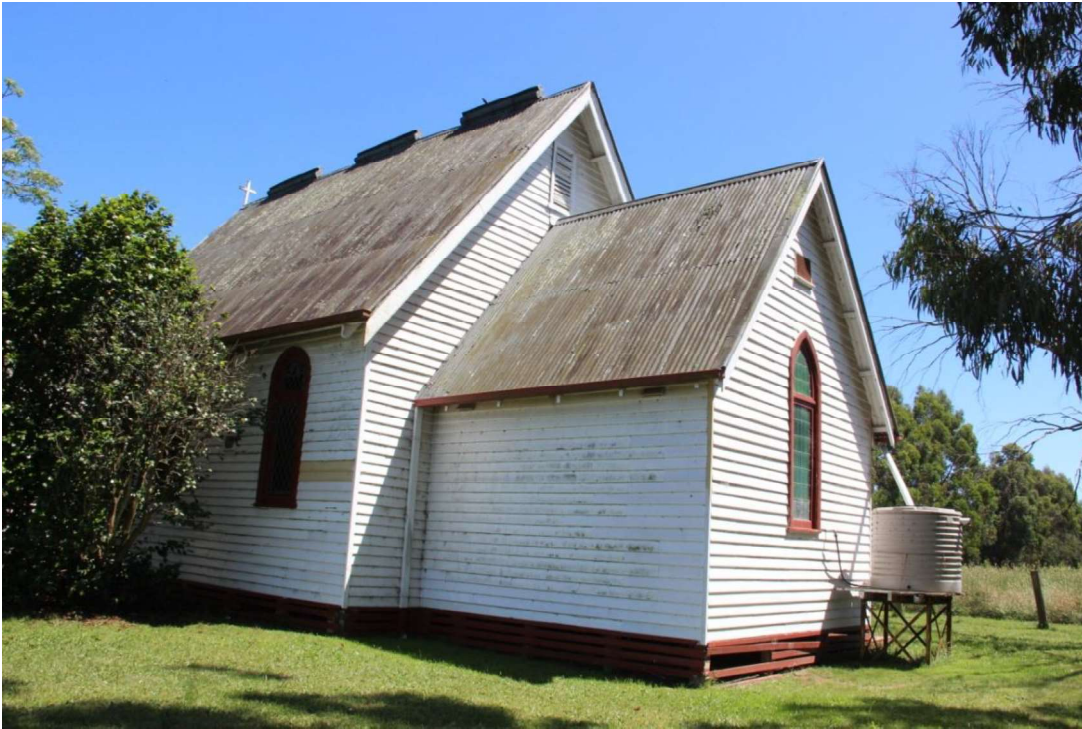
Figure D3. The chancel at the east end of the church is clad in the same weatherboards as the nave of the church, but has a pointed-arch window with simple coloured leadlight. To the left is the camellia, which was donated by a parishioner in the 1950s.
