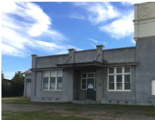
Figure D12. Area D. The south elevation of the 1931 office building. Constructed of brick and rendered, it is divided into three bays with banks of three windows either side of a centrally recessed front door accentuated by the cantilevered porch ‘supported’ by chains attached to the high parapet. The integrity is high however the architectural design is unremarkable compared with the 1908-09 building.
