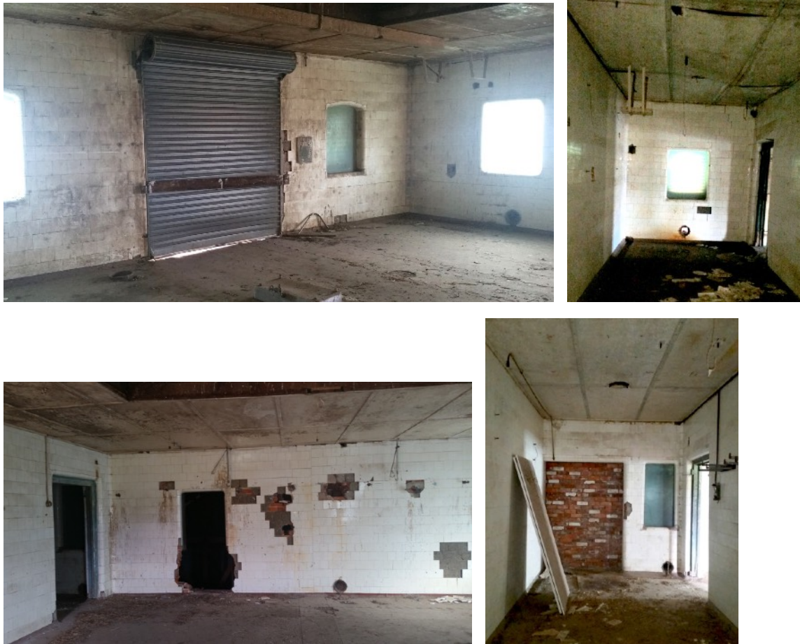
Figure D9. Area H (left) Looking north. Showing the original segmental arched window openings in the north elevation and the square window opening in the east elevation, all with architraves of curved white glazed tiles and white glazed tiles on the walls, and red-brown hexagon tiles on the floor. The roller door is a later alteration. Area I (right) . Looking east to the square window opening, and west to the bricked up opening, with walls clad in white glazed tiles. Note the ceilings may be asbestos cement sheeting. Source. Andrew Martin 2017.
