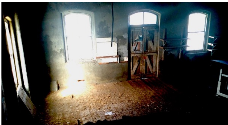
Figure D10. Area J. Looking north, from the loft over area J. Note the intact segmental arched windows, doorway and intact doors. The floor is timber. Source. Andrew Martin 2017.
