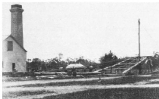
Figure H4. Water tank being erected at Yarram Butter Factory incorrectly dated as 1891 but stack built in 1901. Aylesbury homestead visible in the background. Source. Nicoll, 2008, p. 3
