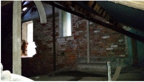
Figure D16, Area K. View towards a former window which has been crudely made into a doorway from Area K into Area H. Source. Andrew Martin 2017.
