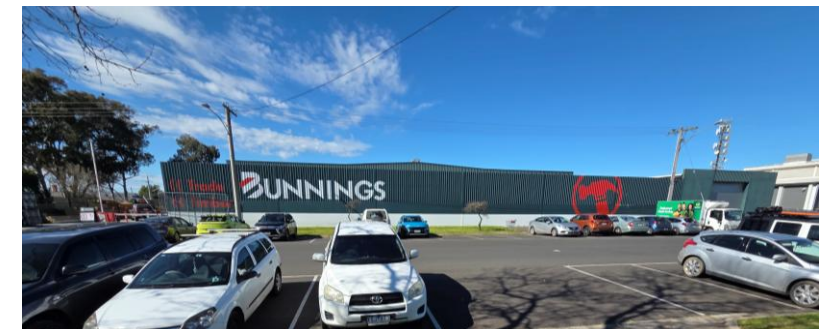
Figure 22: 38-50 Macarthur Street looking east
