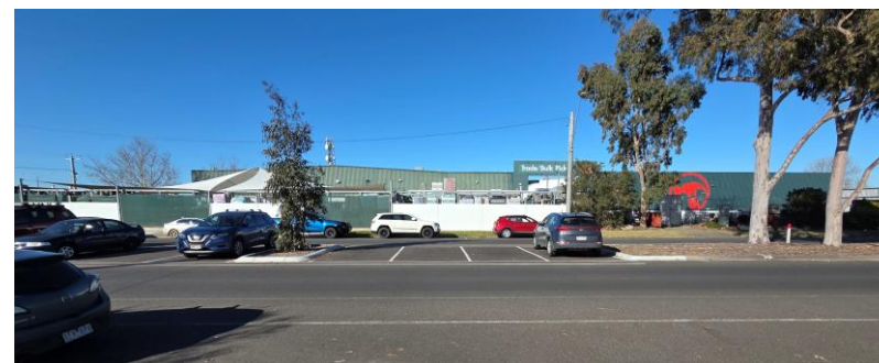
Figure 21: 38-50 Macarthur Street looking south
