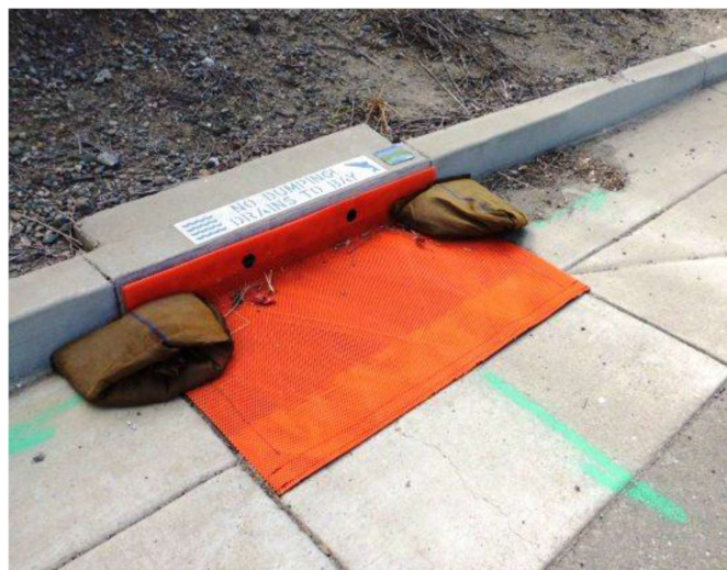
Figure B. Sediment trap (image credit: ERTEC Environmental Systems)
