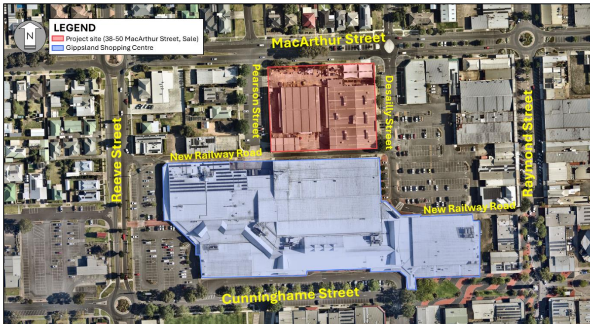
Figure 1: Project Site Aerial (Source: NearMap)
