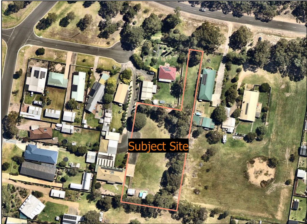
Figure 1: Aerial Photograph of Subject Site (Source: NearMap)
