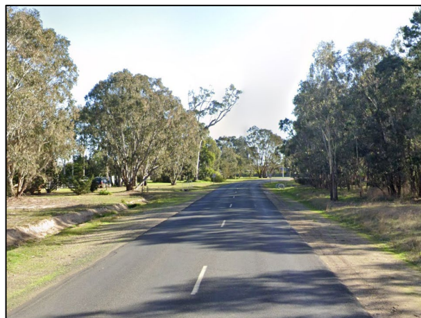
Figure 4: Redbank Rd (view west)
