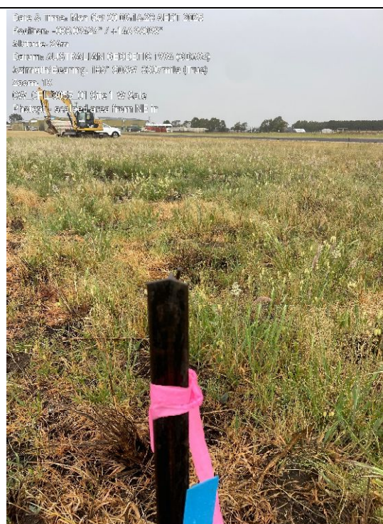
Oct 2025 before scalping: northeast corner looking southwest
