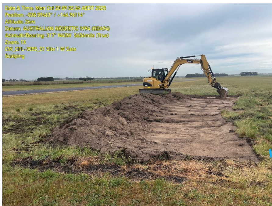
Plate 10. Machine at work scalping
