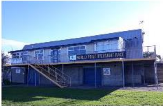
East side and front of Clubhouse
