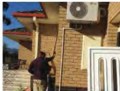
Retrofitting a home gives a better energy rating.
