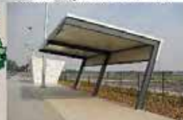
Construction Theme (Building GRSC Netball Shelter)
