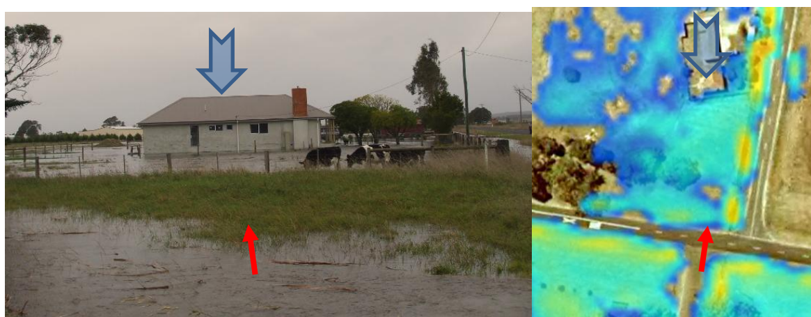
Figure 5-27 June 2012 hydraulic model results compared to photograph from the WSC Rosedale- Corner of Huffers Lane and Willung Road - 5 th June 2012
