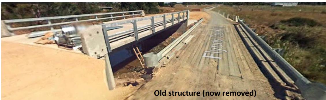
Figure 4-7 Blind Joes Creek – Cansick Street Bridge(s) – April 2008 - Source: Google Maps
