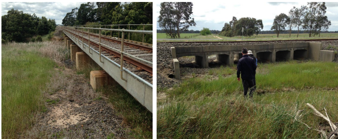
Figure 4-6 Blind Joes Creek – Railway Crossings (West LHS & East RHS)
