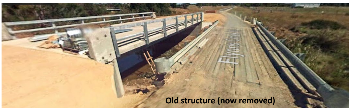
Figure 4-7 Blind Joes Creek – Cansick Street Bridge(s) – April 2008 - Source: Google Maps
