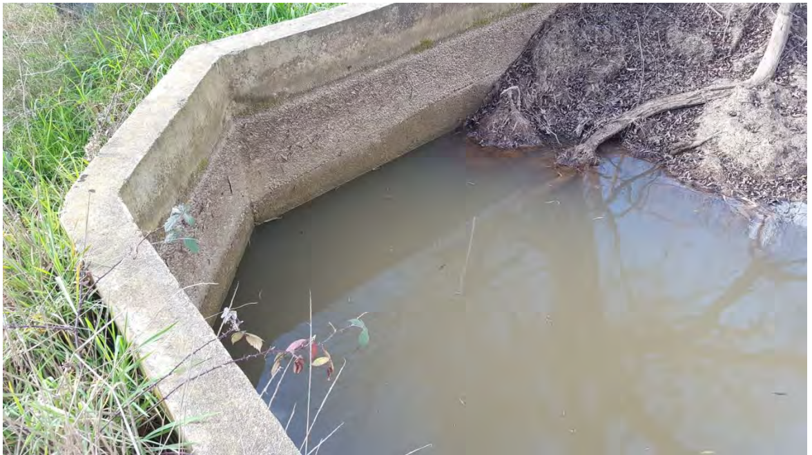
Figure 2.7 Nambrok Denison Drain 4-1 crossing of the Princes Highway
