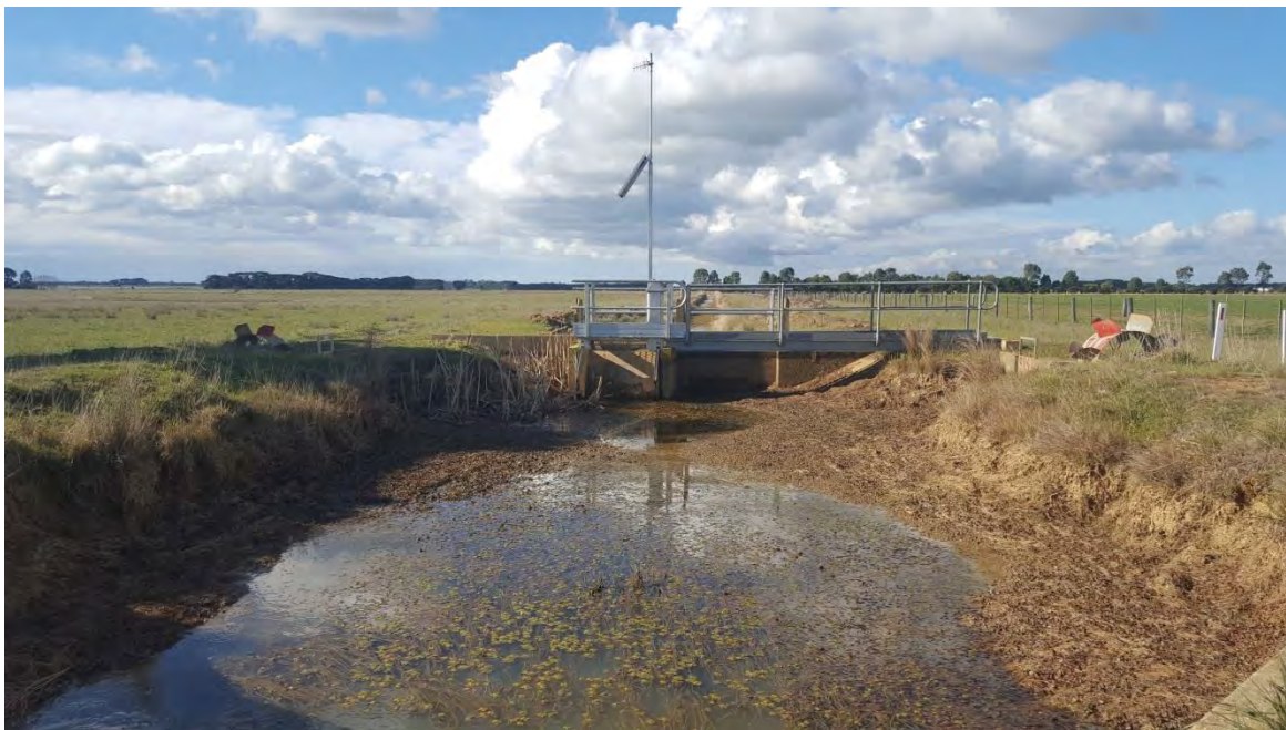
Figure 2.2 SRW irrigation channel and sluice gate at Morris Road
