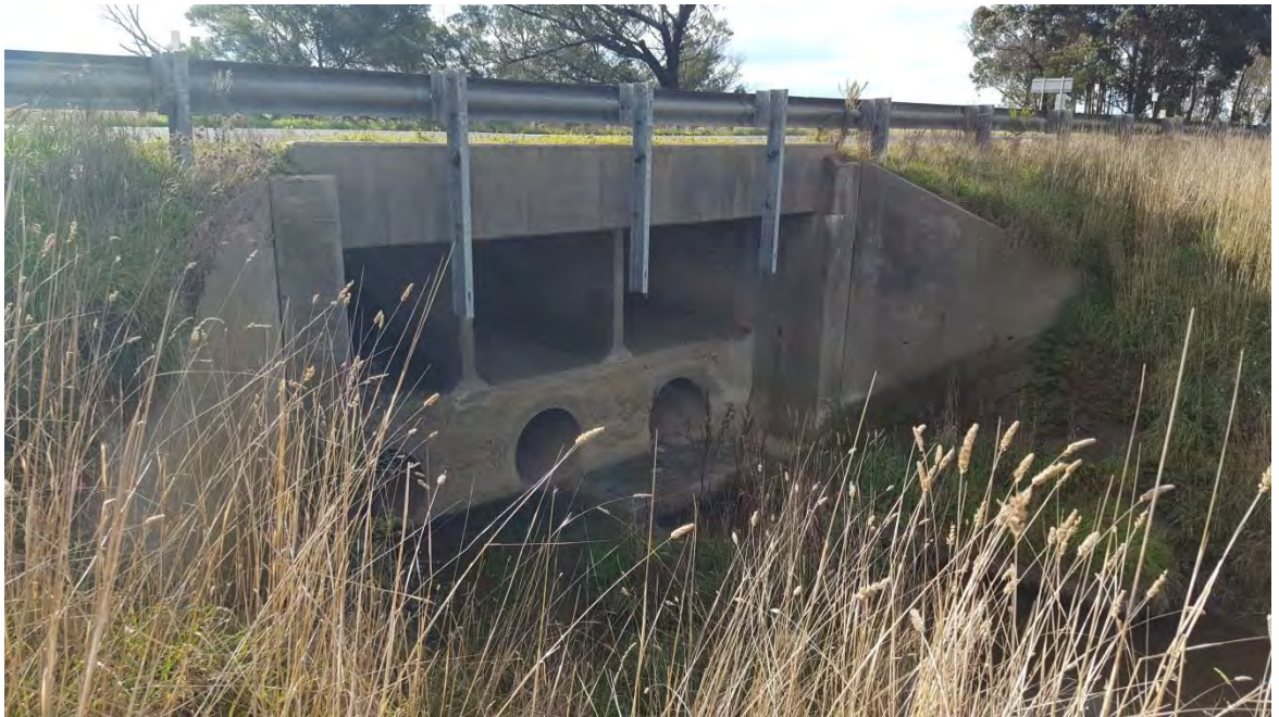
Figure 2.8 Princes Highway crossing on Gippsland Drain No 2 (Nambrok Creek)
