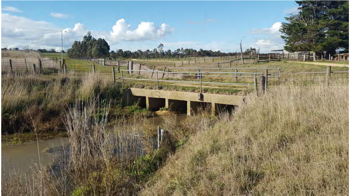
Figure 2.6 Private crossing immediately downstream of the railway on Gippsland Drain No 3
