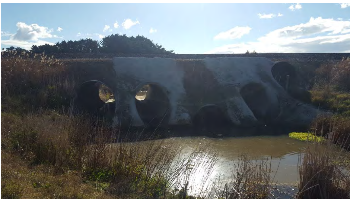
Figure 2.5 Gippsland Drain No 3 crossing at the railway
