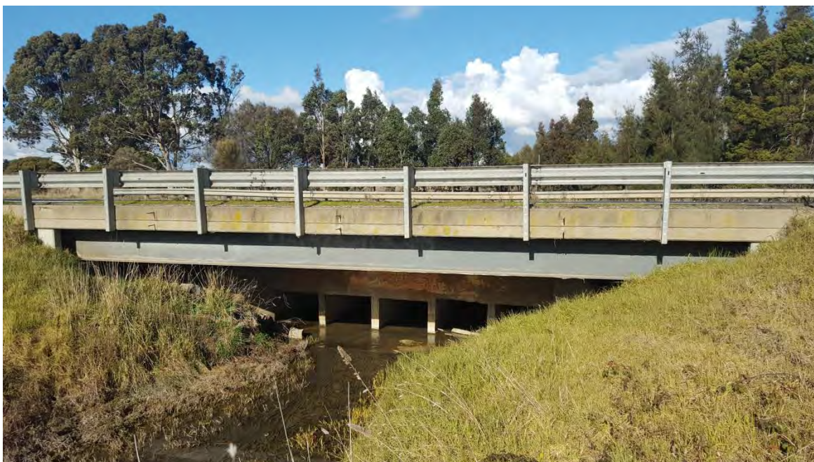
Figure 2.4 Gippsland Drain No. 3 crossing at the Princes Highway
