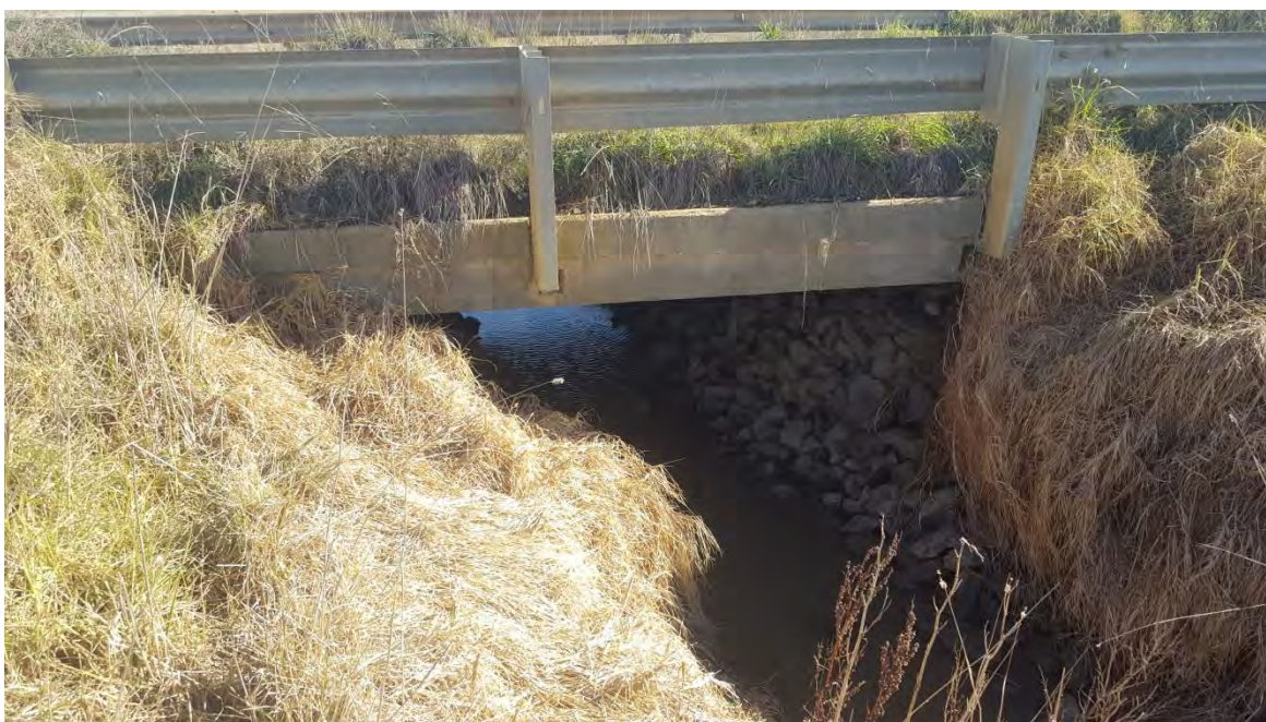
Figure 2.3 Morris Road crossing of SRW irrigation channel
