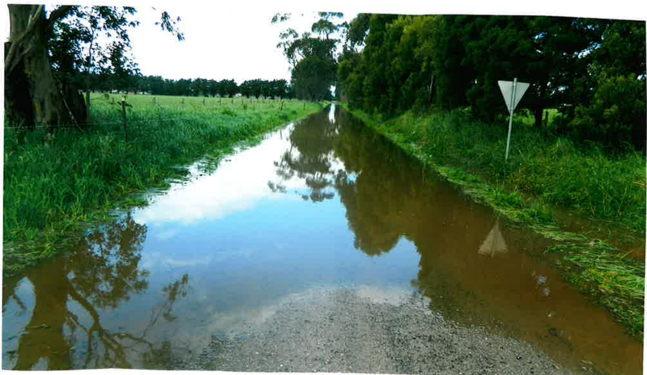
Factory Road / Reserve Road, Yavragon - intersection 2012
