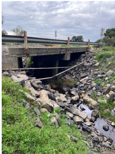
D. Rossiters Road - Nine Mile Creek Bridge
