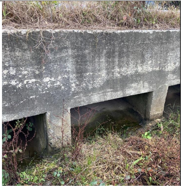
F. Gippsland Highway Box culvert
