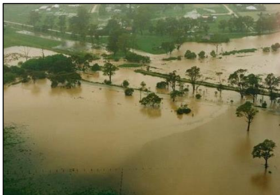
Figure 2 – 1995 Flood Extent -Toongabbie Creek - South side of Township, showing Traralgon-Maffra Road covered by flood waters
