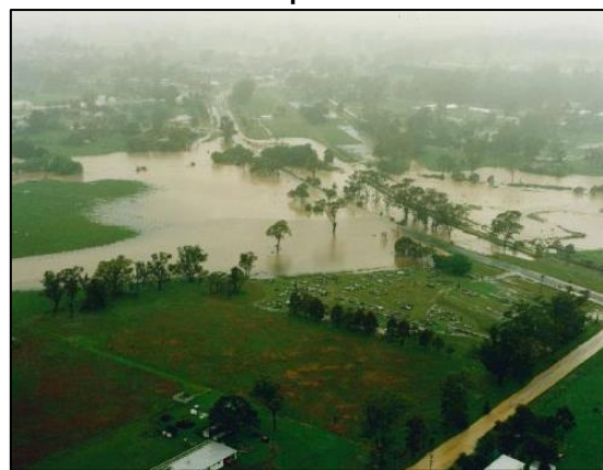
Figure 27 - 1995 Flood Event - Looking north east from Traralgon side showing cemetery in foreground
